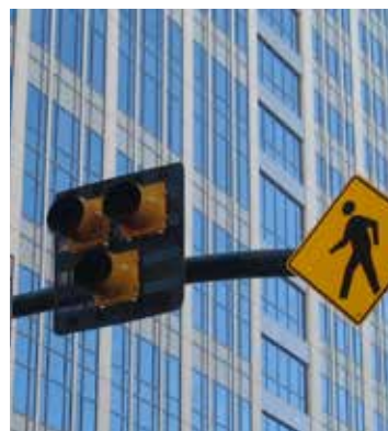
A Pedestrian Hybrid Beacon is a user-actuated beacon that uses amber and red beacons to increase drivers' awareness of pedestrian crossings.
