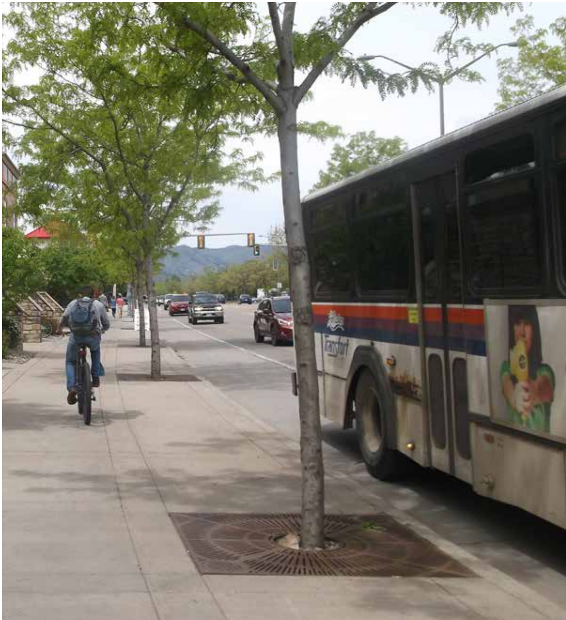
Existing Condition in Campus West
