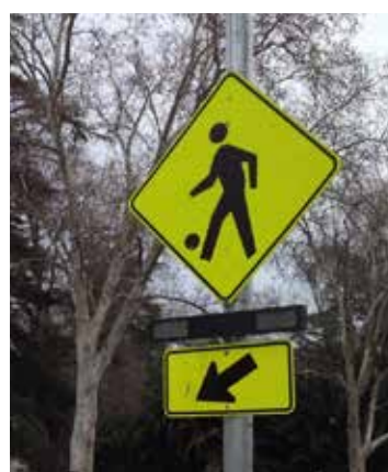
Rectangular Rapid Flashing Beacons are user-actuated amber LEDs that use a flash pattern that is similar to emergency flashers on police vehicles.
