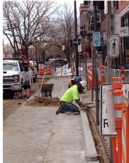
Re-laying brick pavers after concrete replacement
