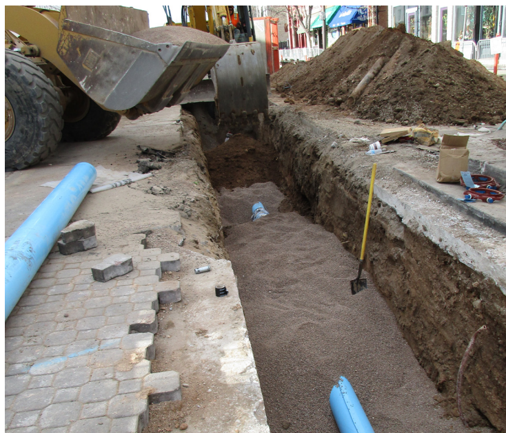
Working carefully around custom pavers for water main installation for tie-in at Linden and Walnut
