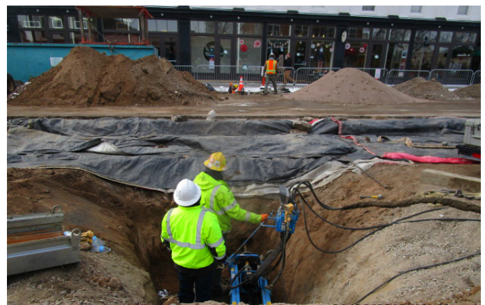
Using boring techniques to install water services and reduce construction impacts
