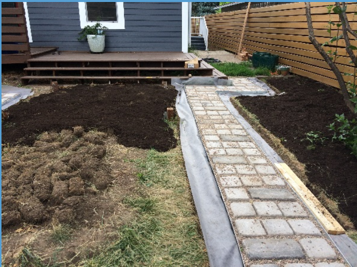
Figure 1: Trench dug alongside pathway and first compost layer.
