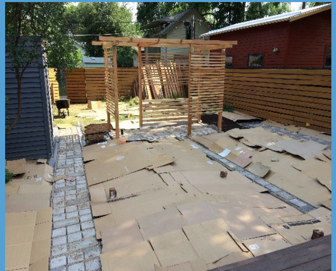
Figure 2: Cardboard layer on top of first compost layer.
