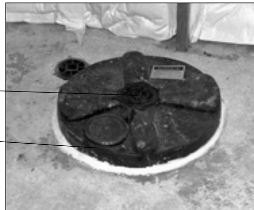
When air is drawn through an unsealed sump cover, it might bring with it radon, other soil gases or moisture.
