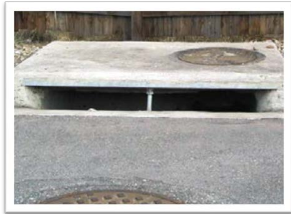
(b) CDOT Type R curb opening inlet
