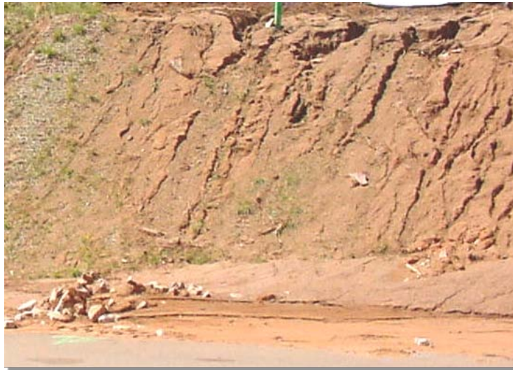
Photograph 7-2. Erosion is a common occurrence during construction activities, which can result in sediment movement off site and deposition in waterways when not properly managed. (Photo courtesy of Douglas County)
