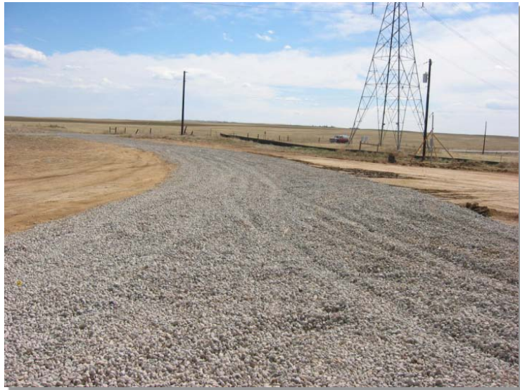
Photograph SCR-1. Stabilized construction roadway.
