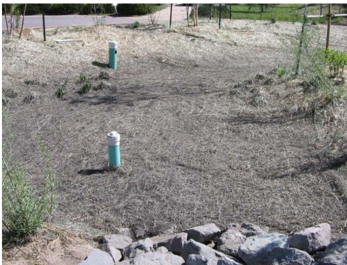
Photograph B-9. This photo was taken during the first growing season of this rain garden. Better weed control in the first two to three years will help the desired vegetation to become established.
