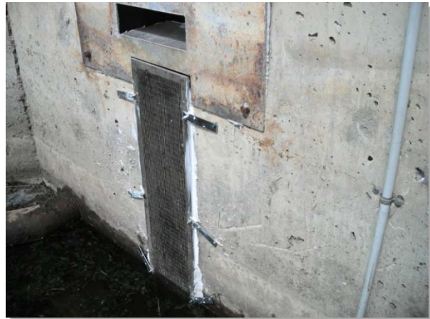
Photograph OS-3. Trash rack after repair.
