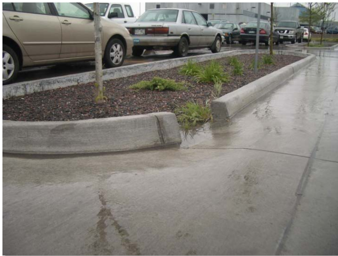
Photograph B-2. The curb cut shown allows flows to enter this rain garden while excess flows bypass the facility. Note: trees are not recommended inside a rain garden
