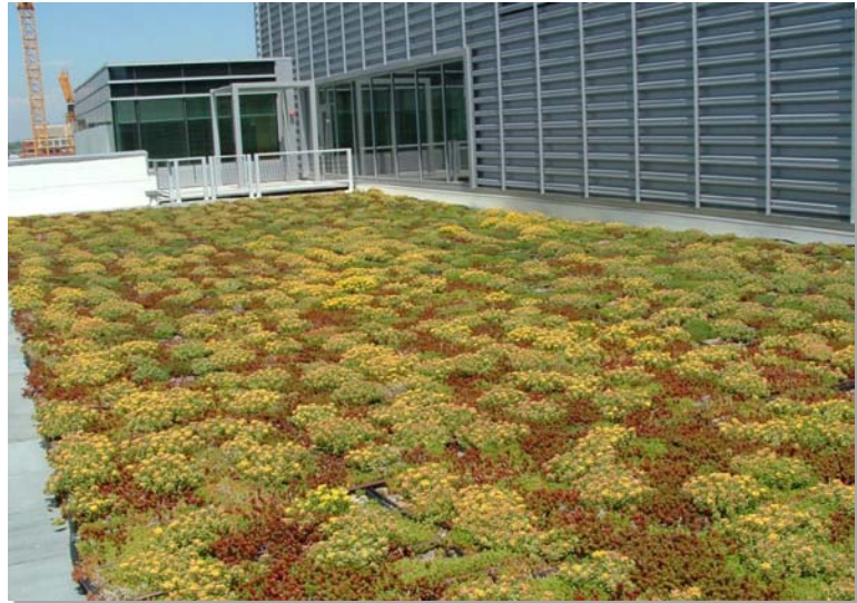
Photograph GR- 4: A modular, extensive green roof in the spring on the Environmental Protection Agency Region 8 Headquarters in downtown Denver. Photo courtesy of Jennifer Boussetot.
