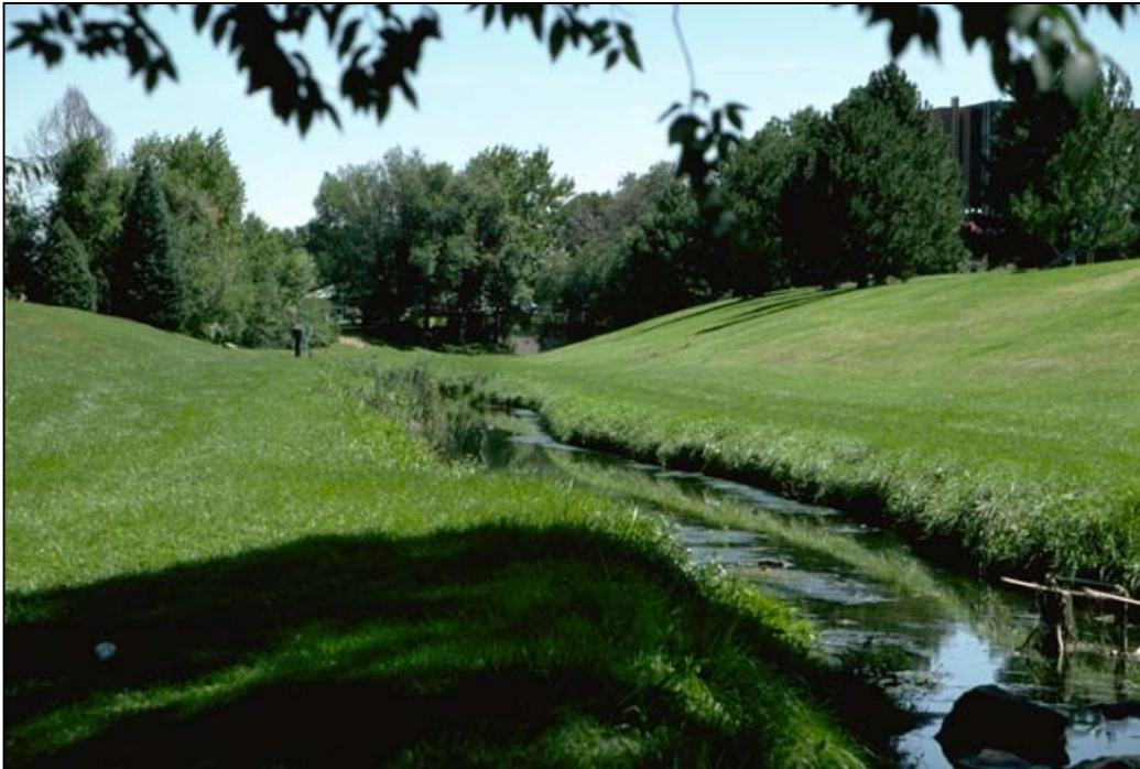
Photograph DP-1—Denver grass-lined channel after 35 years of service. Ann Spirn of the Massachusetts Institute of Technology refers to this channel as "urban poetry" in her publications. Spirn appreciates the soft natural lines.
