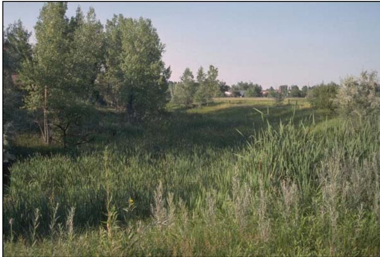
Photograph DP-4—Drainageways having “slow-flow” characteristics, with vegetated bottoms and sides can provide many benefits.
