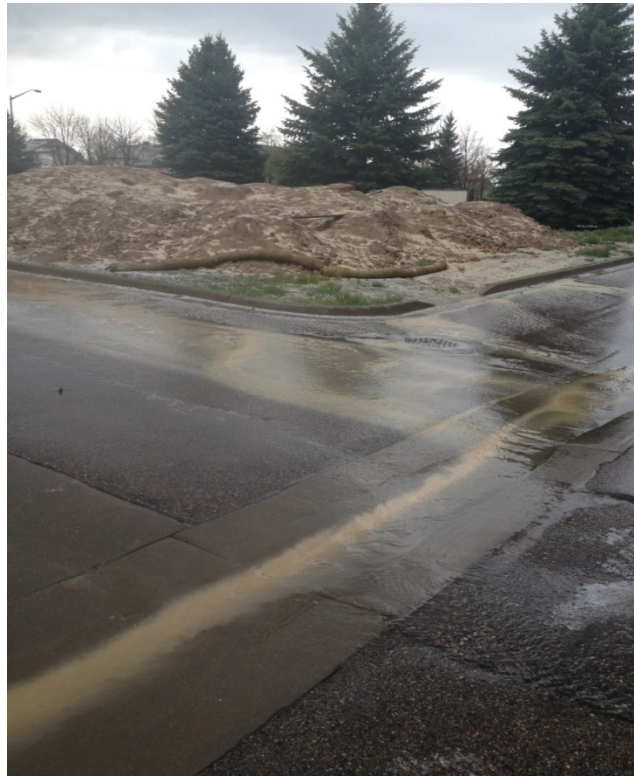
Improperly installed Best Management Practices on a small construction site caused discharge of sediment.
