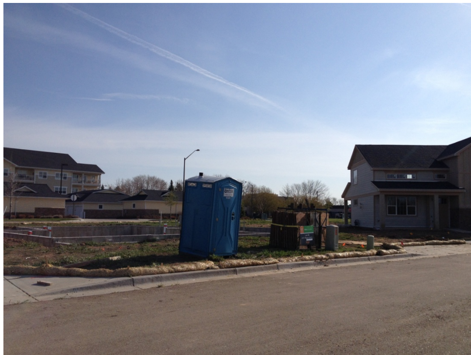
Straw wattles and staked portable toilet on construction site.
