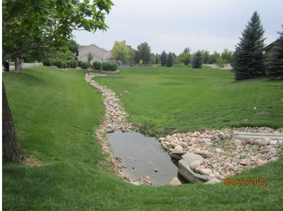
Stormwater basin after required inspection and maintenance were completed.
