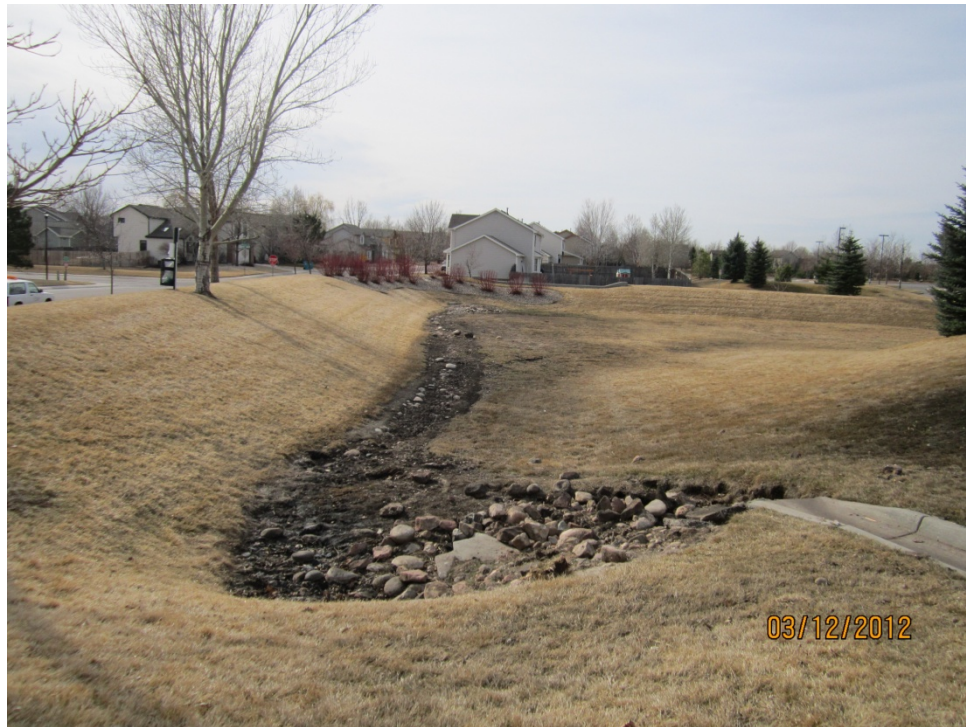
Stormwater basin before inspection and required maintenance were completed.
