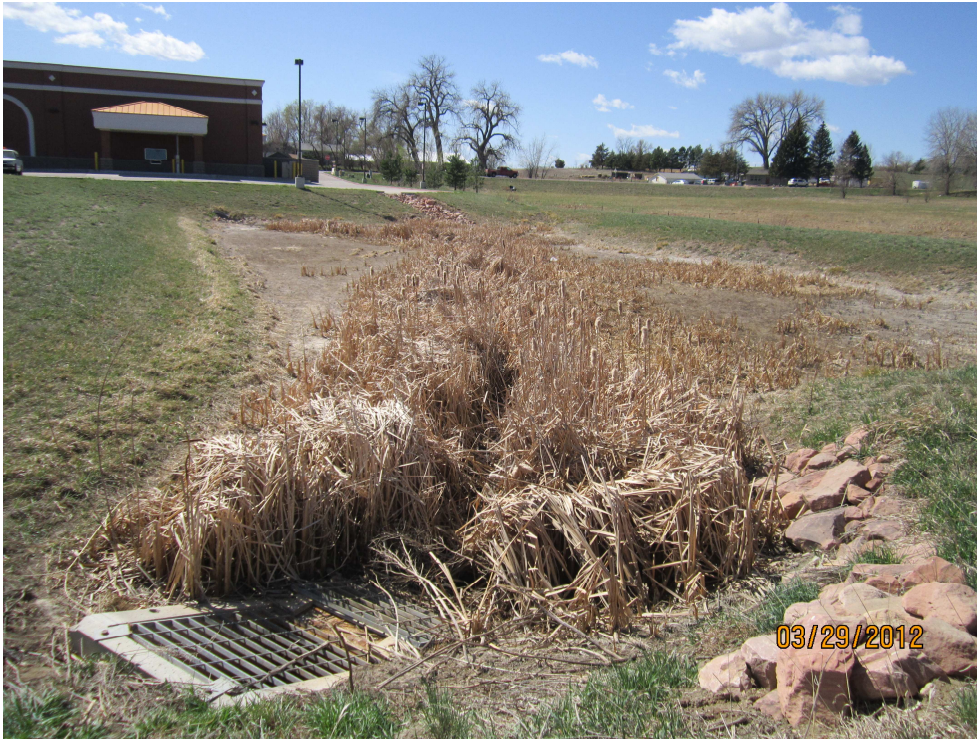
Water quality swale not functioning properly due to needed maintenance
