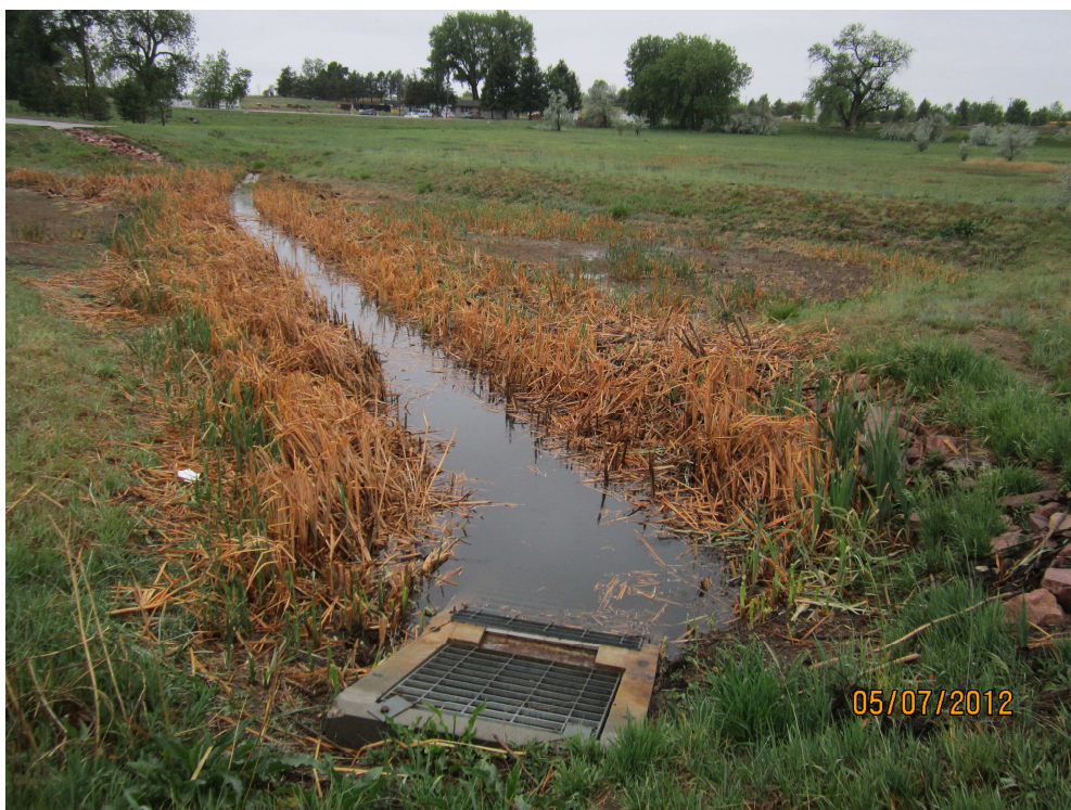
Properly functioning water quality swale after maintenance was performed
