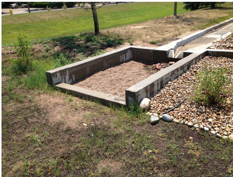
Utilities Service Center Bioretention pre-Treatment Forebay, June 2012
