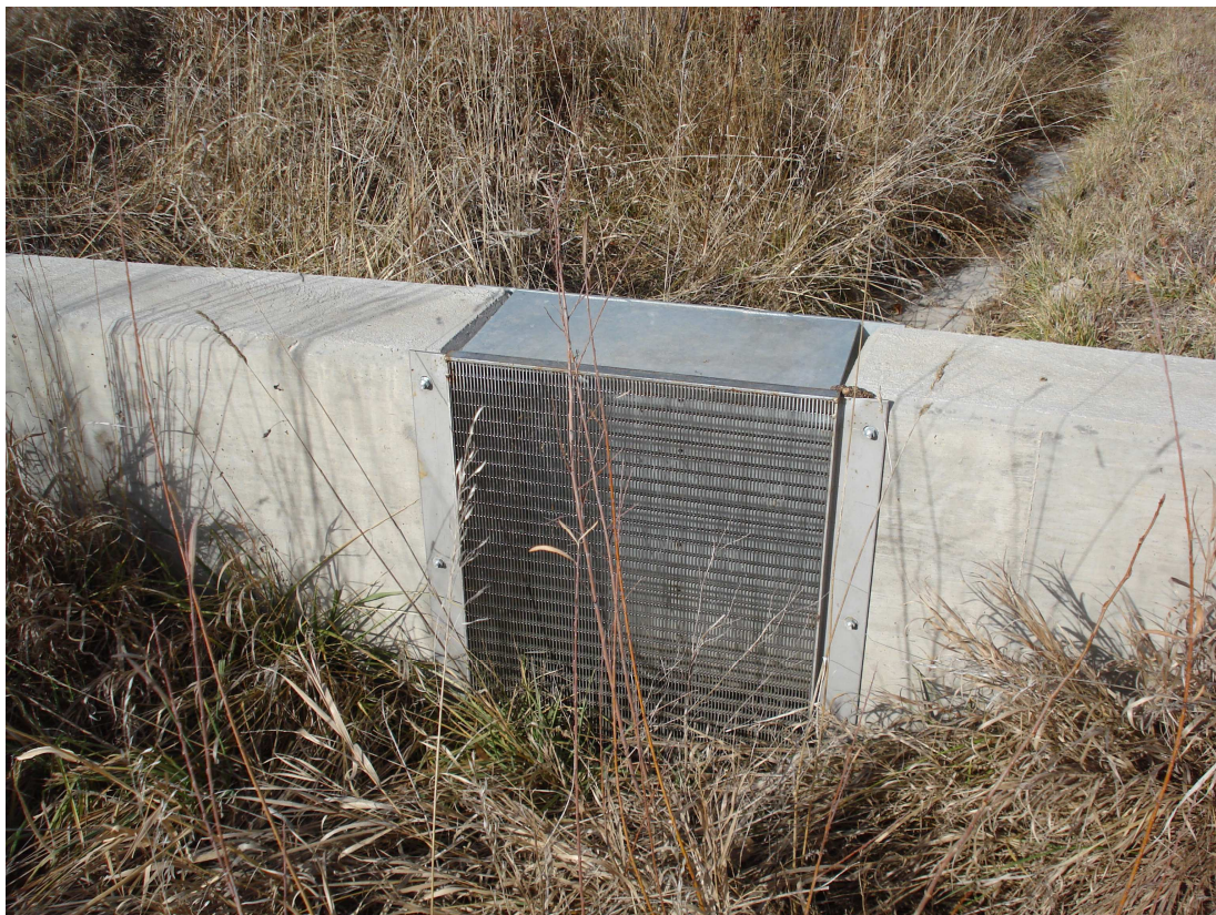
Water quality weir helps remove pollutants from stormwater
