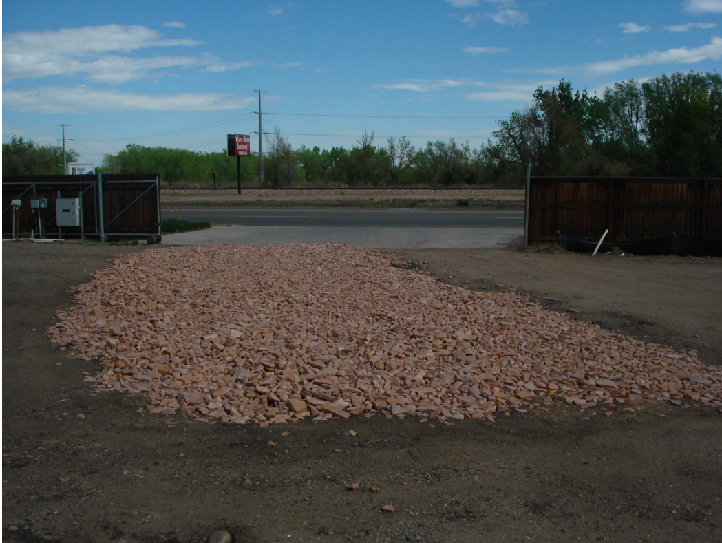
Vehicle tracking pad help prevent construction vehicles from tracking mud onto the street
