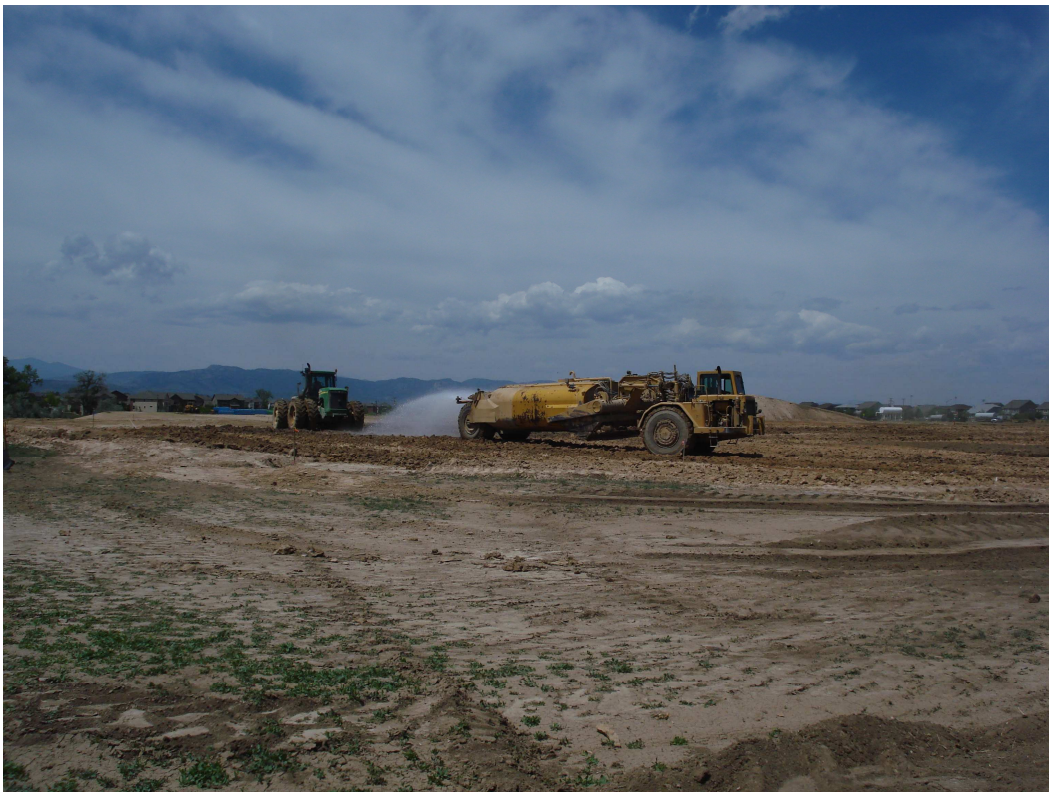
Construction site watering operations help reduce wind erosion
