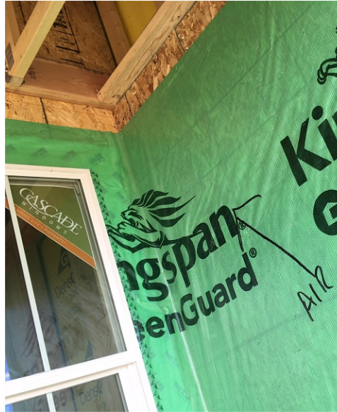
Exterior front porch looking at porch roof.
