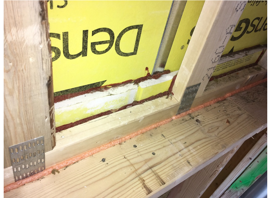
Top plate from above – 6" ripper filling the gap is visible
