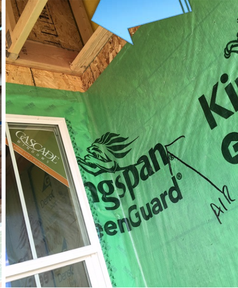
Exterior front porch looking a porch roof.
