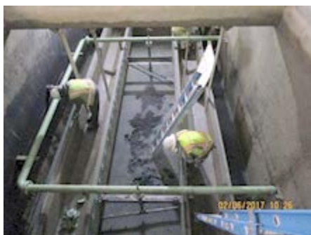
Inspecting a filter underdrain
