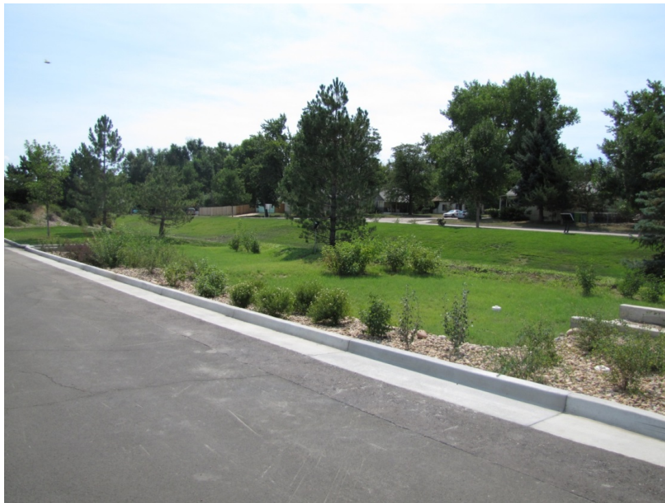
Bioretention Cell completed landscape.
