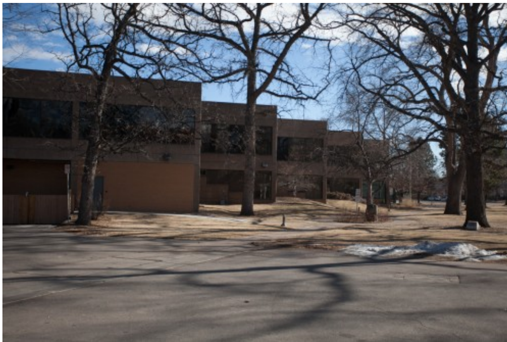
Library Park Parking Lot (Before Rain Garden Installation)
