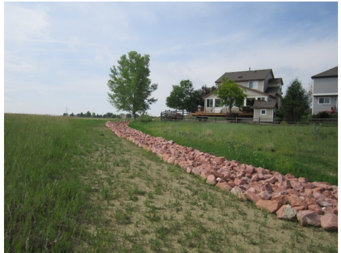
This channel was repaired by re-grading the area, installing rip rap and vegetating with native seed.
