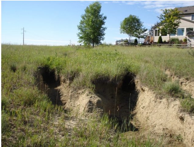
High Velocity stormwater flows caused erosion of this channel into a wetland detention basin.
