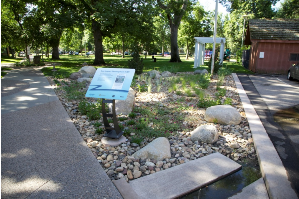
Library Park after Rain Garden Construction
