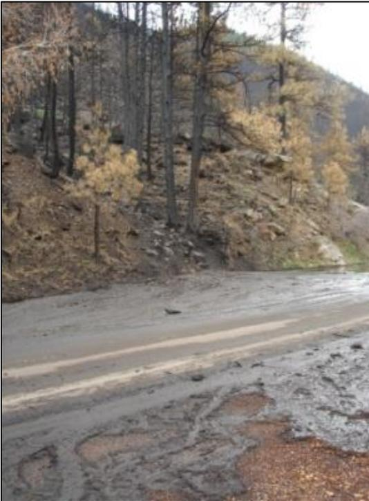
**Figure 8.** Debris flow across Highway 14 in the High Park burn area following a rain event during summer of 2012.
