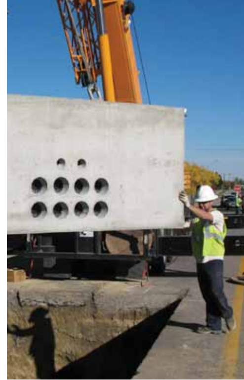
Portner Substation construction.
