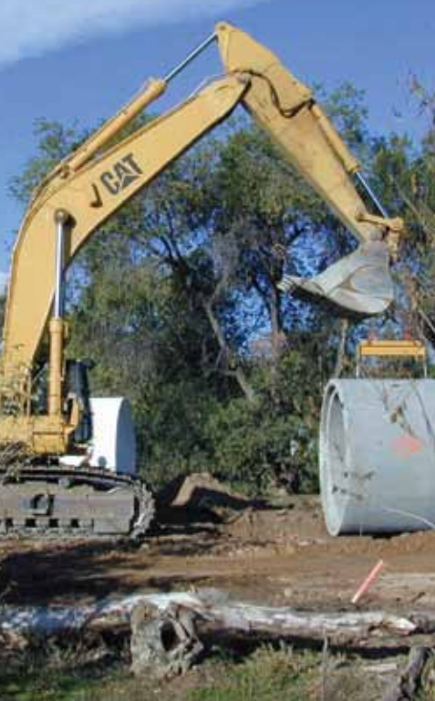
Stormwater improvement project.
