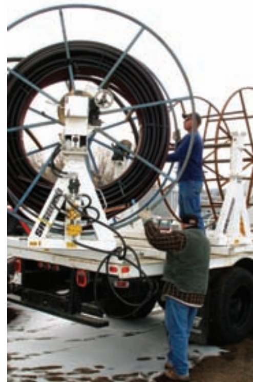
Unloading electric cable.
