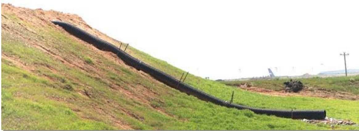
Photograph TSD-1. A temporary slope drain installed to convey runoff down a slope during construction. Photo courtesy of the City of Aurora.
