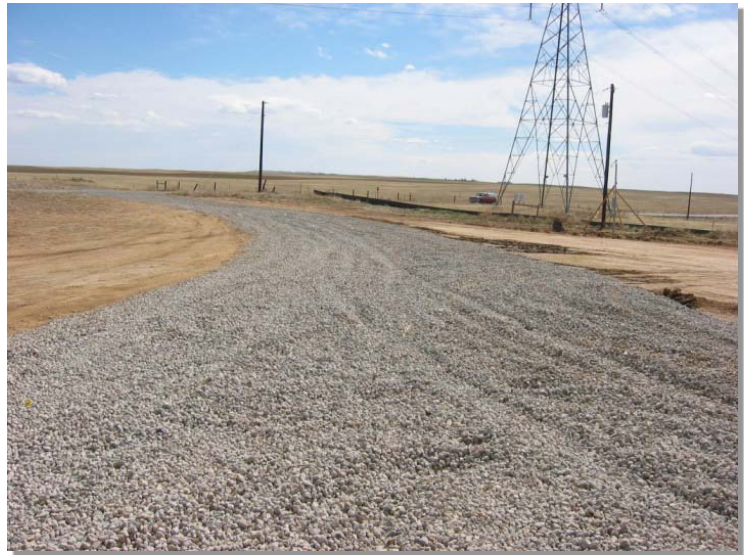
Photograph SCR-1. Stabilized construction roadway.
