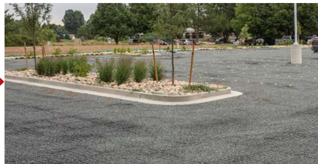
Gravel Grid Pavement Example
