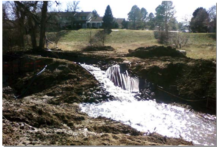
Photograph TDC-1. Use of a temporary diversion channel (right side) to enable installation of a grade control structure (left side). Photo courtesy of WWE.
