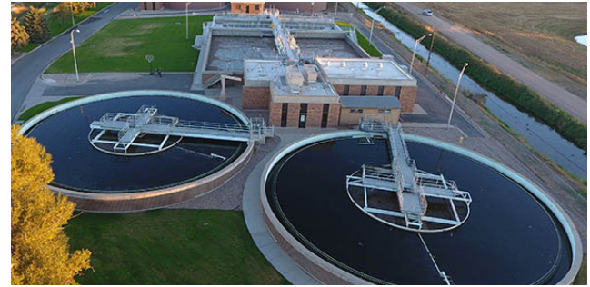
Aerial view of the Drake Water Reclamation Facility, which treats about 23 million gallons of wastewater per day.
