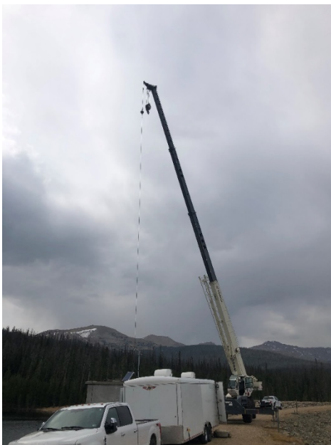
Crane on top of dam used to lower men into work area, 120'
