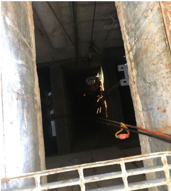
Going down into the shaft.
