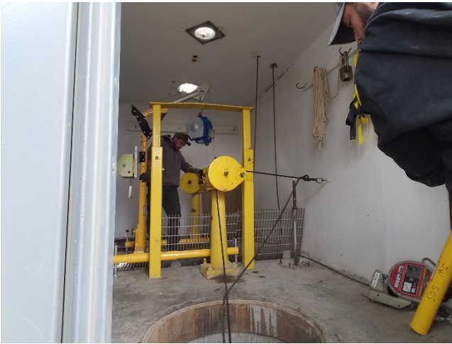
Above ground, lowering basket.
