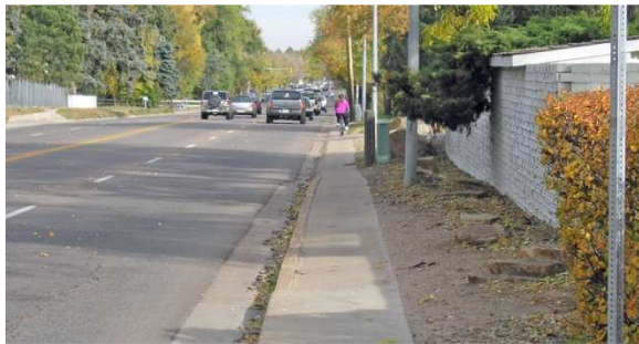
Example of a constrained arterial (East Prospect).
