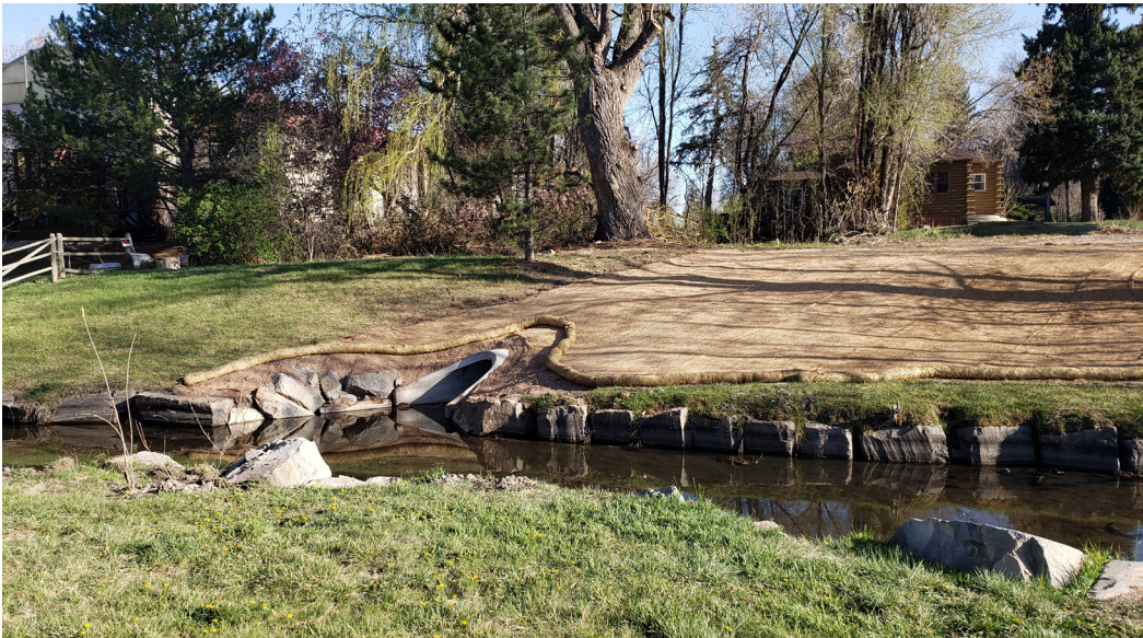
Left: A new storm pipe enters Spring Creek just downstream of Remington Street. Above: Revegetation phase of the Stover and Stuart Street Stormwater Outfall Project, completed in 2022.
