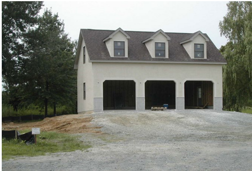
Figure 22: Three-Car Garage Elevated on Fill
