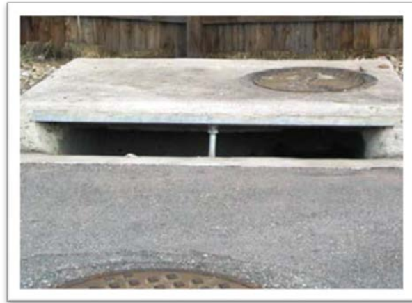
(b) CDOT Type R curb opening inlet
