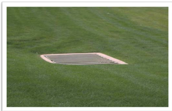
Photograph 3.6-2. Inlets frequently need maintenance.
