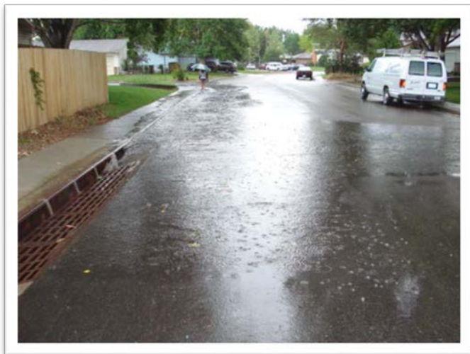
Photograph 3.4.2-1. Weir performance decay can be observed in this picture as flow appears to enter only the first two inlets while exceeding the height of the upstream curb.
