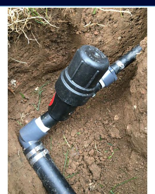
Install pressure reducer and wye screen combination filter to lateral line
