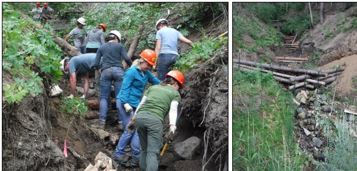
Figure 5. Project partners and volunteers work together to stabilize the Unnamed Tributary-3 drainage
