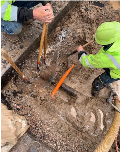
Figure 15 – Repairing a main leak
