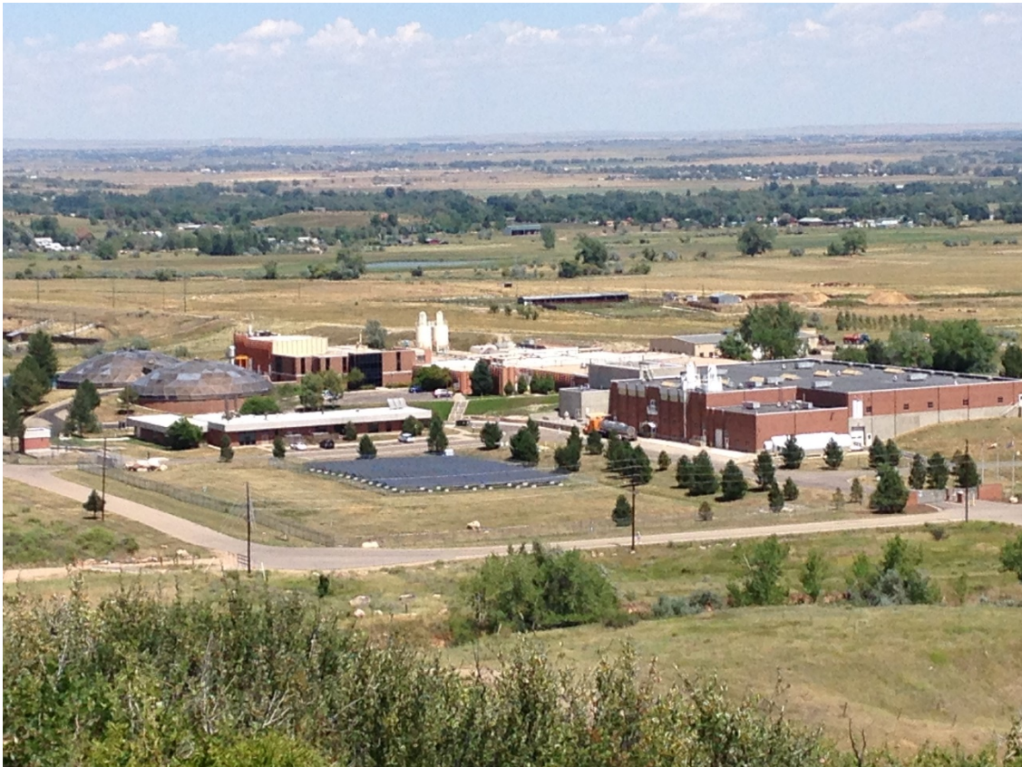
Fort Collins Water Treatment Facility
