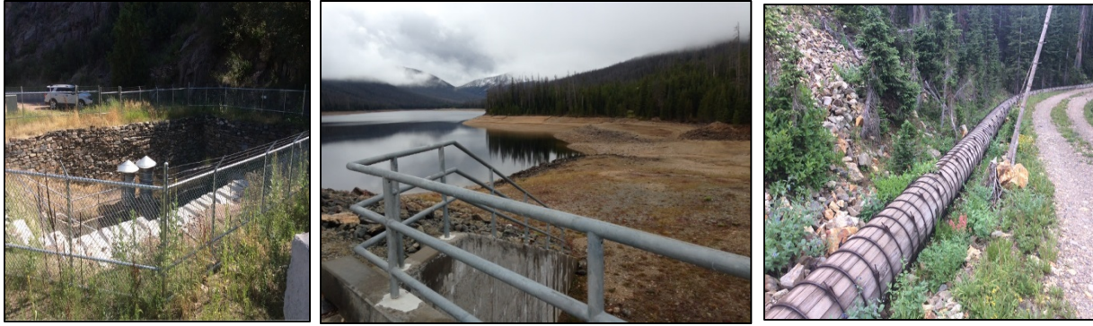
Figure 8. Photos show a diversion tunnel, reservoir and section of pipe that were evaluated as part of the Drinking Water Infrastructure Wildfire Risk Assessment.
