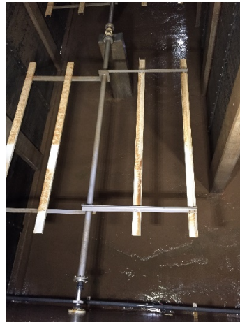
Figure 12 - Flocculator
