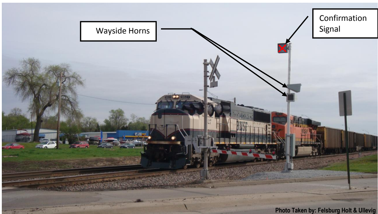
Figure 15. Highway-Rail Crossing Equipped with Wayside Horns
