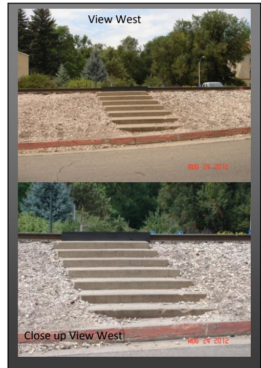
Figure 12. Ped Crossing #2 at BNSF
