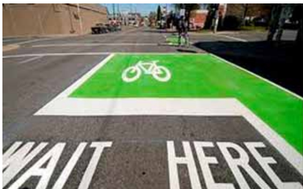
A bike box is a colored area at a signalized intersection that allows bicyclists to pull in front of waiting traffic.
