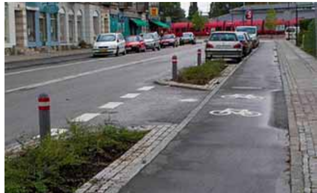
Properly designed cycle tracks reduce conflicts between bicycles and parking cars by placing the cycle track on the inside of the parking lane.
