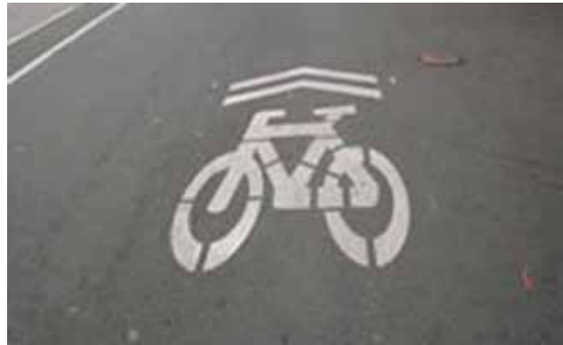
Shared Lane Markings provide a reminder to share the travel lane and encourage bicyclists to "take the lane."
