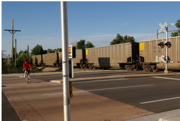
The Mason Trail currently crosses Harmony Road at-grade, adjacent to the BNSF Railroad crossing.
