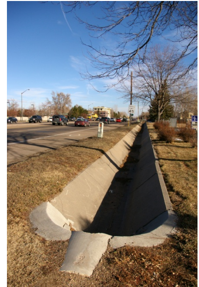
The abandoned concrete-lined ditch on the south side of Harmony Road, just east of College Avenue.
