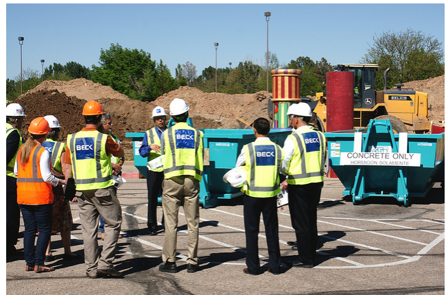
Foothills Mall reconstruction recycled 76% of the material generated by the project.
