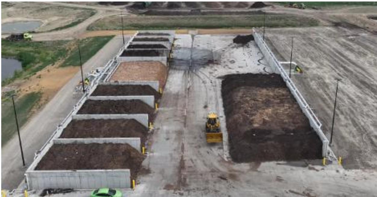
Figure 16: Engineered Compost Systems (ECS) example of a 20,000 TPY ASP Curbside Food Scrap and Yard Trimming Facility
