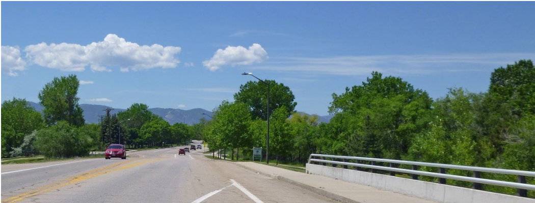
Example of a landscape-dominated stretch of an entryway corridor.
