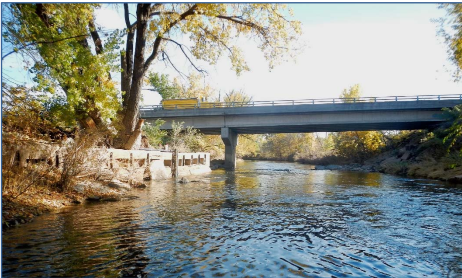
Figure 2.49 Historic Concrete Structure Obstructing the Upstream Side of the Lincoln Avenue Bridge
