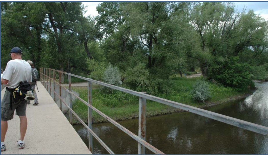
Figure 2.11 McMurry Pedestrian Bridge, Note Non-Compliant Railing
