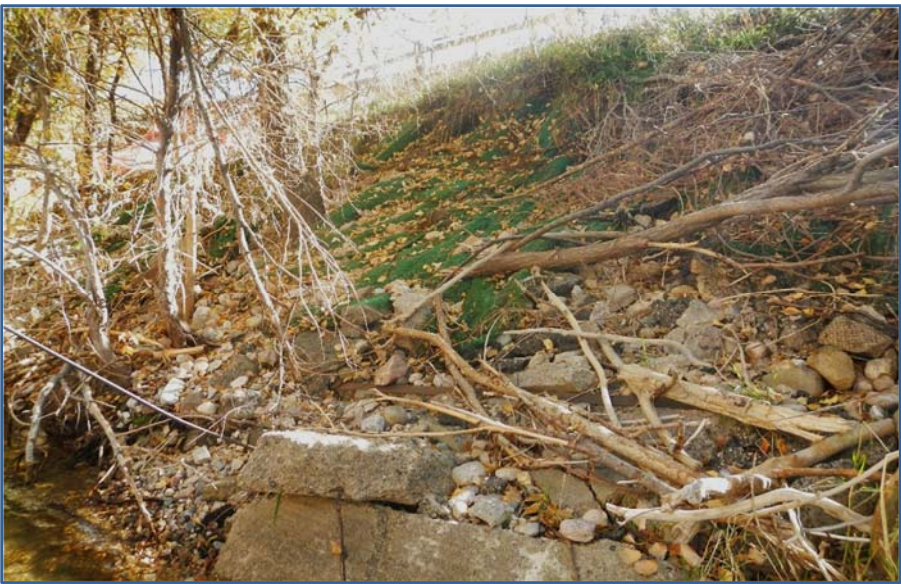
Figure 2.35 Bank Erosion, Concrete Rubble, and Exposed Plastic Turf Mat on South Bank, West of the BNSF Railroad
