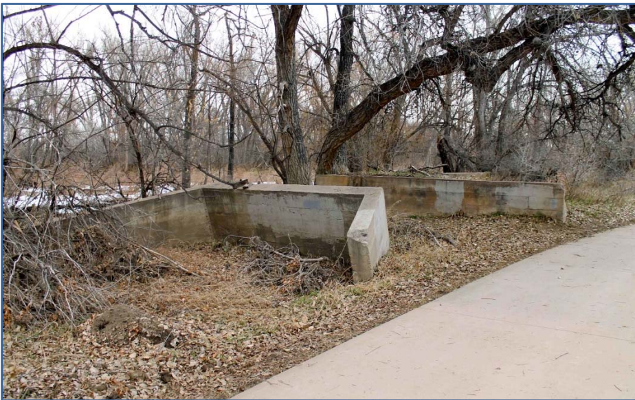
Figure 2.9 Historic Mason & Hottel Mill Race Headgate Structure
