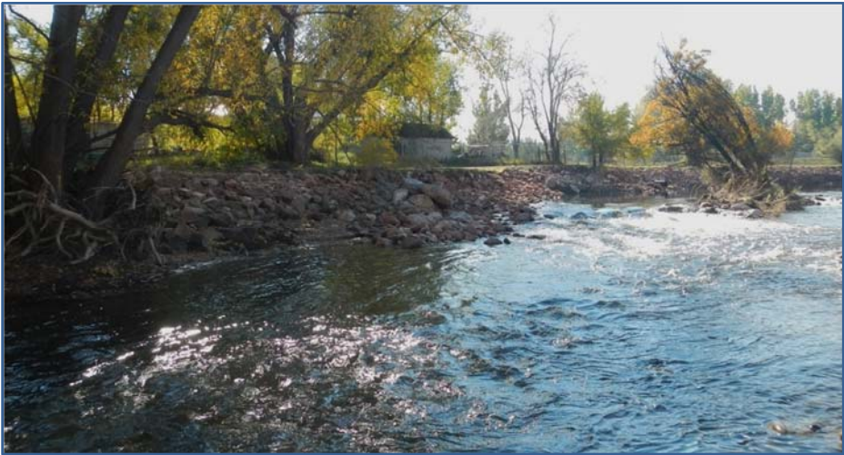
Figure 2.6 Exposed Riprap Bank Armoring near Wood Street
