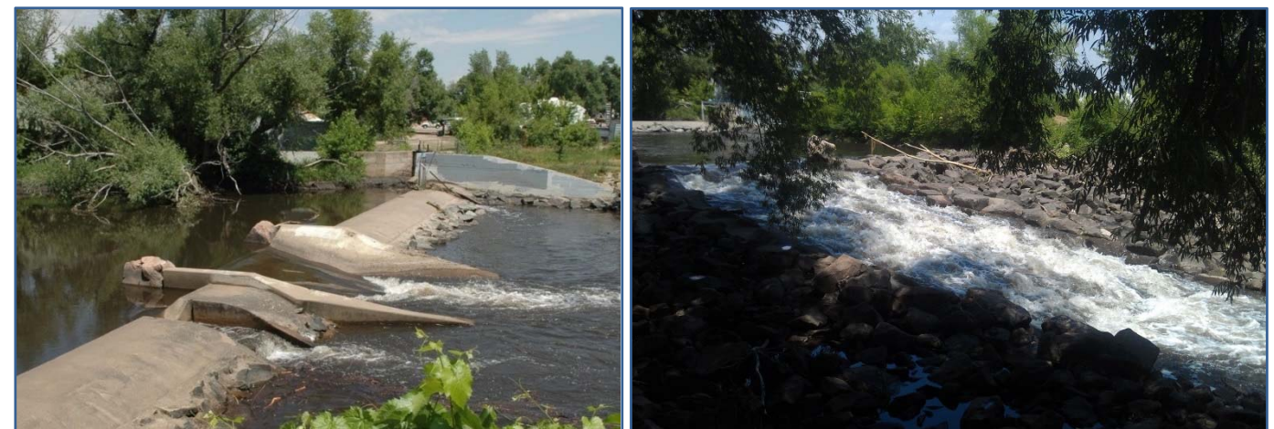
Figure 2.31 Coy Diversion Structure (left photo), Boat Chute (right photo)
