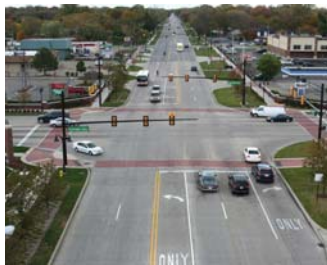
Crosswalk at intersection
