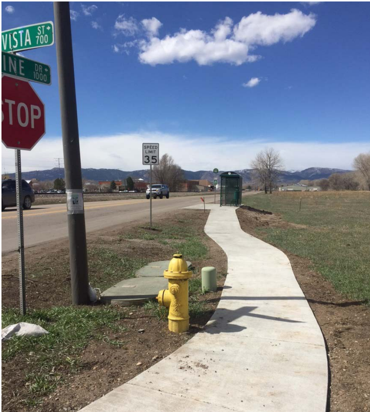
Alta Vista/Vine Drive – New sidewalk to bus stop, new bus shelter
