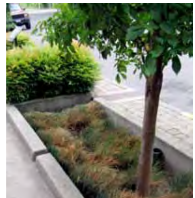
This ROW planter area allows water from the street and the sidewalk to be channelled into it.
