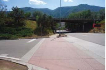
Colored Concrete Crossing in Glenwood Springs, CO
