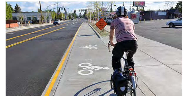
Pavement markings at this driveway crossing on the Cully Street Cycle Track in Portland, Oregon notify cyclists and drivers of a potential conflict area.
