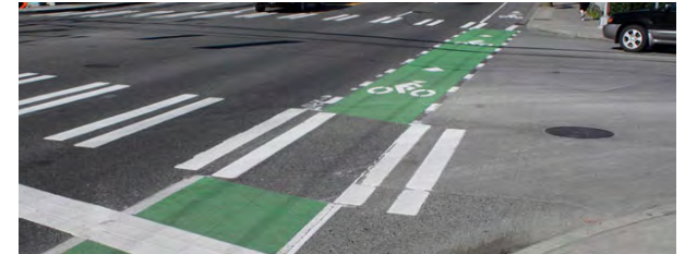
Colored pavement at intersections & driveways increase the visibility of the facility and identifies areas of conflict.
