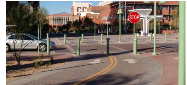
Colored concrete pavers increase the visibility of a shared-use path crossing a roadway in Tucson, Arizona.
