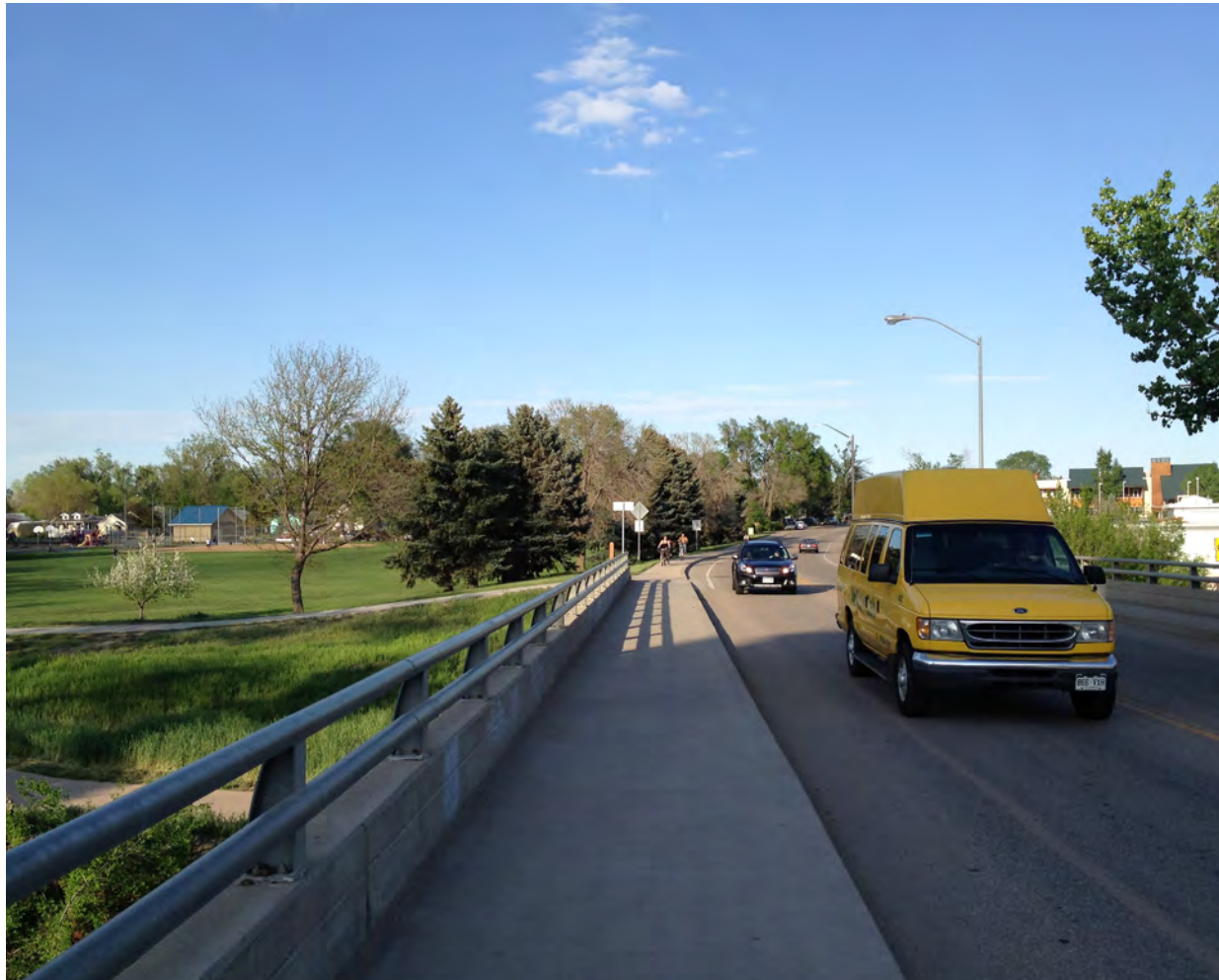
Lincoln Corridor Bridge
