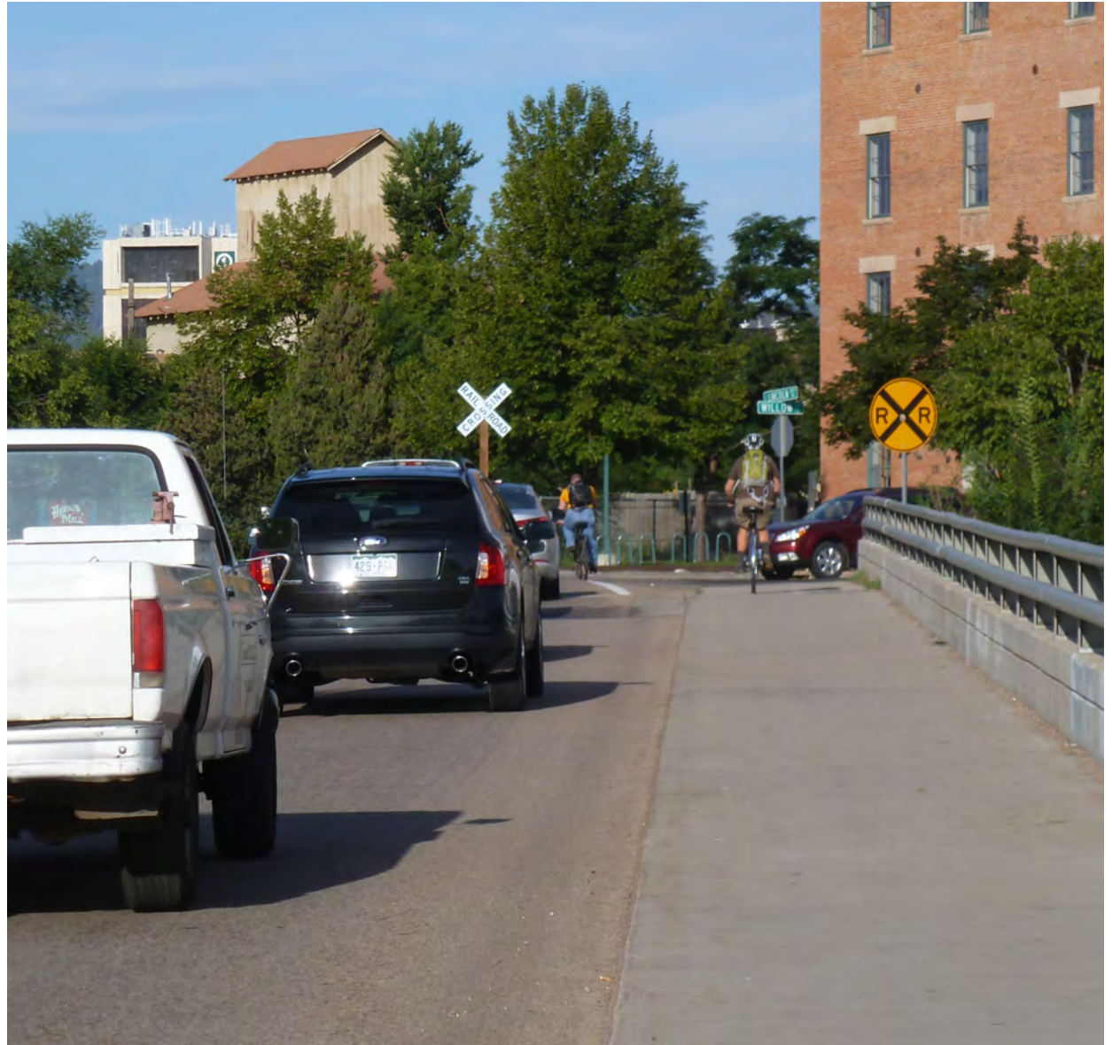
The Lincoln Bridge
