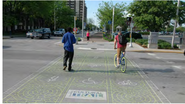
A crosswalk in Indianapolis, Indiana provides dedicated space for users of a Share-Use Path at a roadway crossing.
