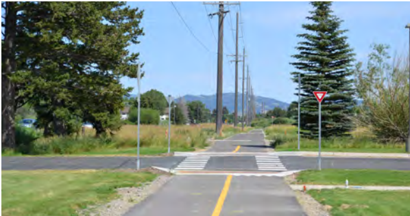
“Elephants feet” treatment increases the visibility of a shared-use path as it crosses a roadway in Billings, Montana.
