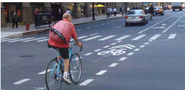
Dotted lines and shared lane markings guides bicyclists through the intersection in a straight and direct path.
