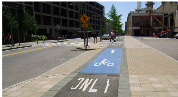
Driveways crossings are a unique challenge of protected bike lane design. Color is used to identify the conflict area along this Cambridge, Massachusetts bike lane.
