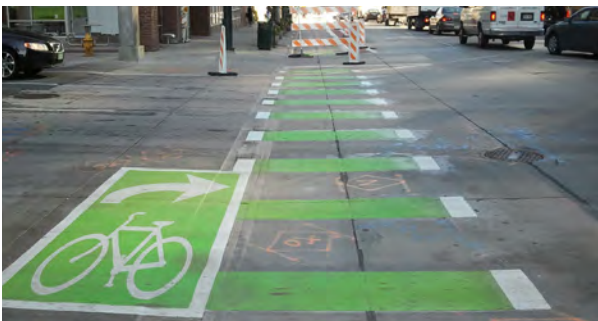
Intersection crossing markings in Denver, Colorado raise awareness for both bicyclists and motorists to potential conflict areas.
