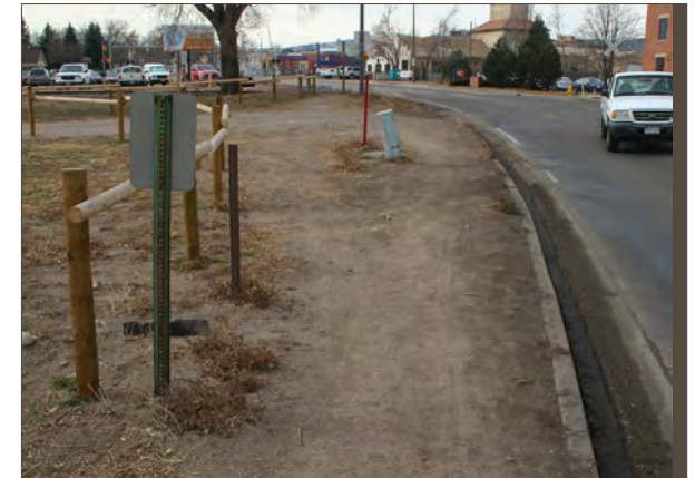
Sidewalks are lacking along much of Lincoln Avenue.
