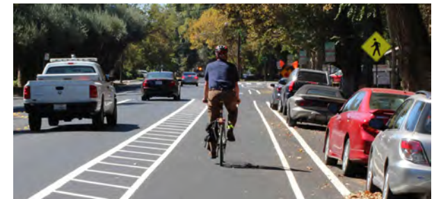
A "dual" buffered bike lane in Davis, California provides cyclists separation from both parked and moving cars.
