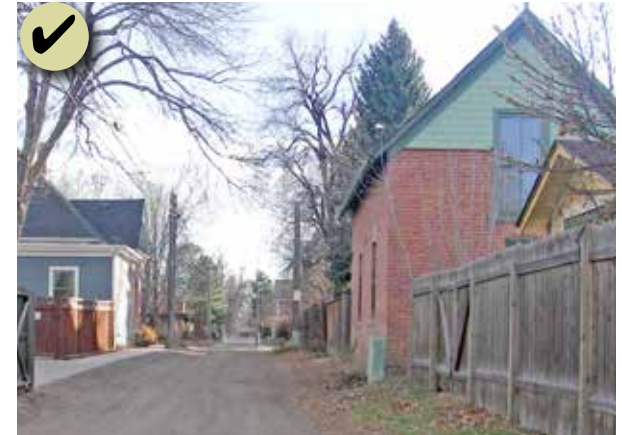
Figure 119: This one-and-a-half-story carriage house is oriented with the roof plane parallel to the alley. This building has been appropriately preserved.
