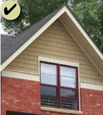
Figure 162: The combination of brick and wood material is appropriate; brick is typically the base material and wood is used as an accent.
