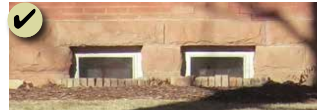
Figure 114: Maintain and repair a historic foundation.
