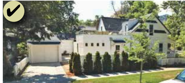
Figure 171: This addition steps down from the historic building, is a contemporary design, uses complementary materials and is a subordinate mass.
