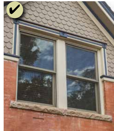
Figure 67: This reconstruction of a historic window maintains the significant features and stylistic elements that were present in the original construction of the building.
