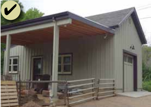
Figure 177: Design the mass, form and roof shape of a new accessory building to be compatible with the primary building and surrounding historic context.
