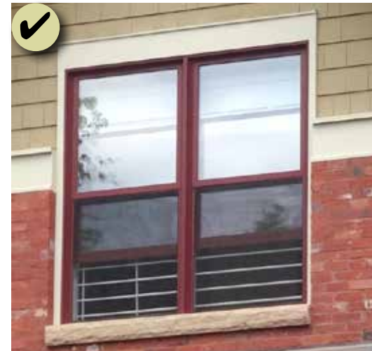
Figure 158: When using contemporary window patterns and designs, ensure they respect the character, alignments and proportions of windows in the surrounding historic context.
