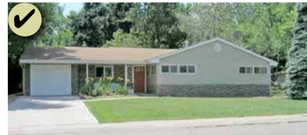
Figure 190: Traditionally, most parking was accessed from alleys in the neighborhoods; however, Character Area 6 reflects a development pattern where much of the parking access is off of the street leading to an attached garage.
