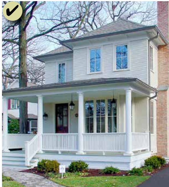
Figure 134: Design a building to be compatible with the context. A hip roof, simple building form and raised porch are appropriate features on this building. Porch and eave height are scaled appropriately.
