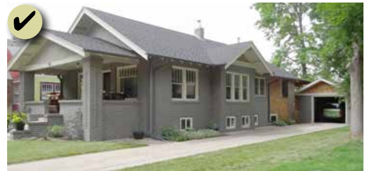
Figure 174: Differentiate an addition from the original structure with an offset and change in material.
