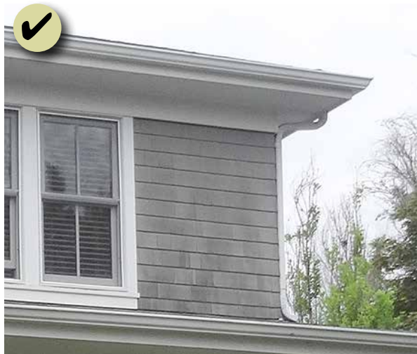
Figure 169: Boxed eaves with generous overhangs are appropriate.
