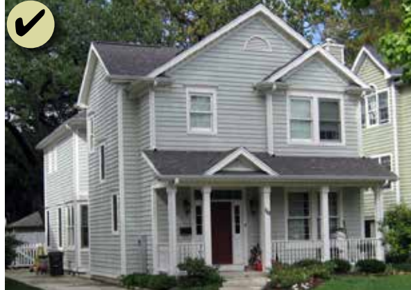
Figure 133: This building has several compatible features such as the traditional massing, porch, articulation and materiality.
