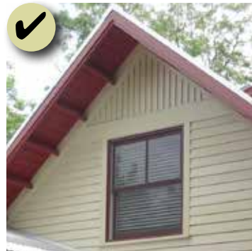
Figure 165: This combination of horizontal and vertical wood siding is an appropriate application. Note how the vertical boards highlight the gable end in a unique design approach.
