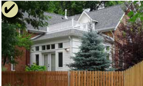
Figure 172: Differentiate an addition from the original structure with an offset and change in material.
