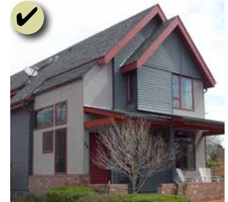
Figure 144: This contemporary building applies appropriate vertical and horizontal articulation techniques along the front and side wall planes.
