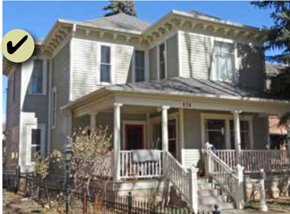
Figure 111: A hip roof with boxed eaves and brackets tops the primary form, and a hip roof form tops the porch.
