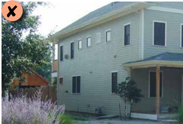
Figure 145: This building wall is inappropriate; it is too long and does not have any wall offsets.
