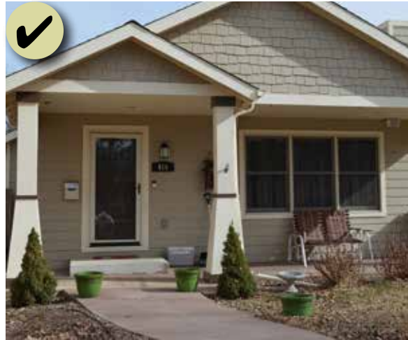
Figure 151: Use a front porch to define the entry. This porch uses Craftsman detailing.
