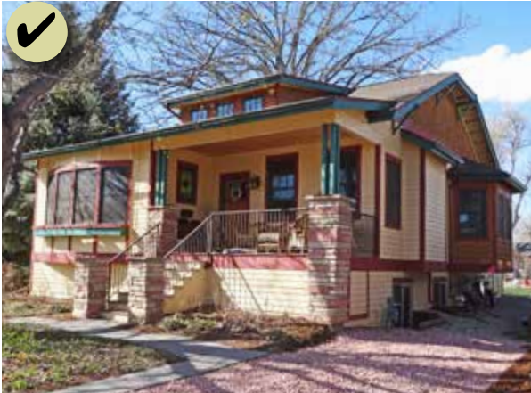
Figure 109: Clipped, side-gable roof form with loft dormer
