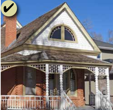
Figure 62: Retain and treat exterior character-defining features and examples of skilled craftsmanship with sensitivity. Important features include turned columns, upper porch spindles and zipper brick corners.
