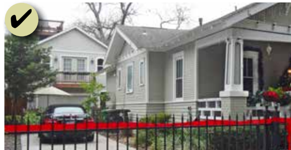
Figure 173: Use simplified version of building components and details found in the surrounding historic context on additions, such as the arched windows and deck detailing on this addition.
