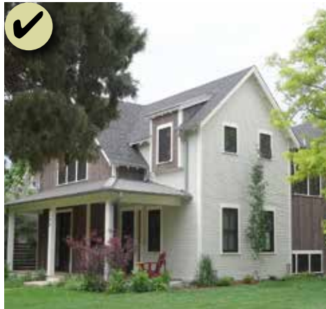
Figure 140: Use façade articulation techniques to help a building fit within the scale of the surrounding historic context.
