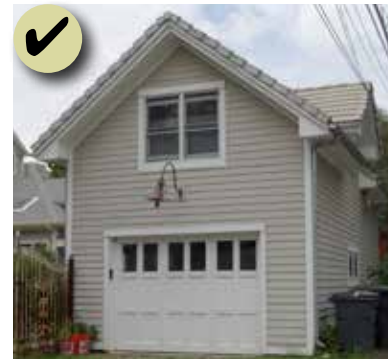
Figure 181: This new accessory building with a living unit above may be too large for most contexts; however, it is a compatible scale for some historic contexts.
