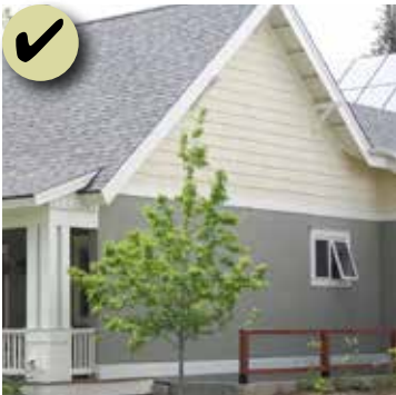
Figure 164: The combination of stucco and wood material is appropriate. In this example stucco is the base material with a wood accent in the gable. The reverse is also appropriate.
