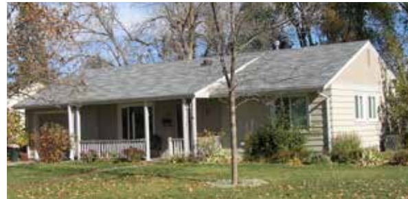
Figure 53: Character Area 6 Ranch with porch front addition
