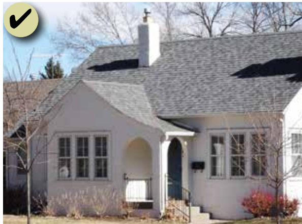
Figure 112: A gable roof with shallow eaves tops the primary form and a splayed gable roof form tops the one-story projecting entry feature.
