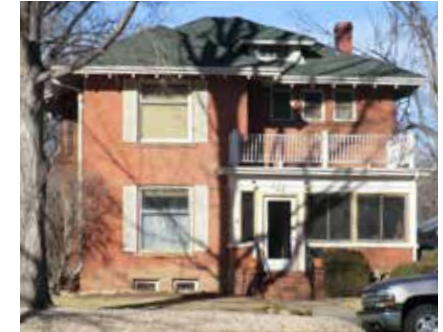
Figure 9: Character Area I Vernacular with an altered porch and Craftsman detailing at the eave
