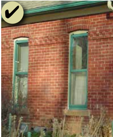
Figure 80: Repair and weatherization is often more energy efficient, and less expensive, than replacement.
