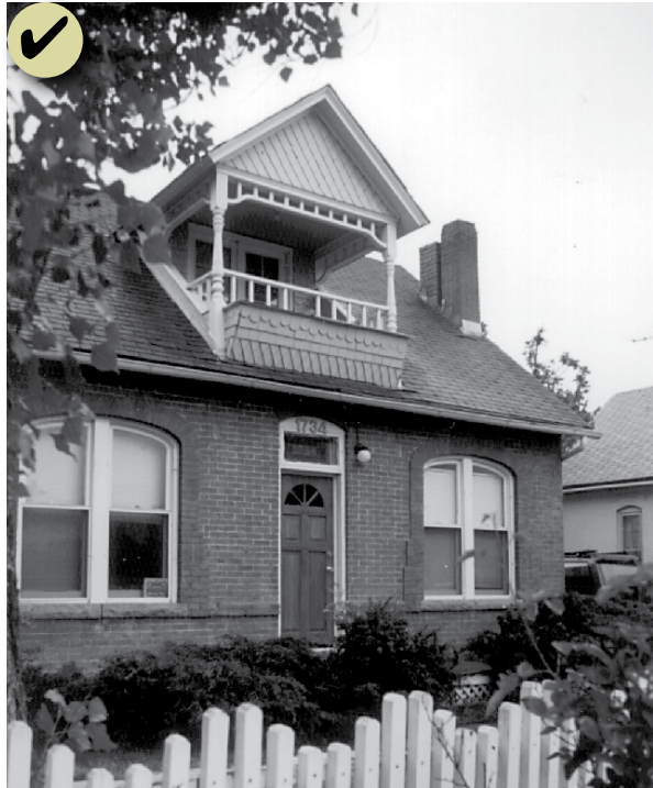
Figure 149: A small balcony may be appropriate on the front of a new building if it is modest in size and incorporated into a gable end or porch roof.
