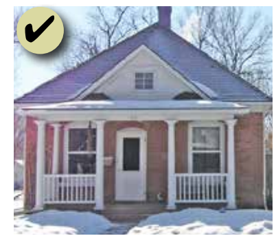
Figure 101: A porch is one of the most important character-defining features of a façade.
