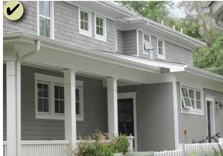
Figure 143: Use façade articulation techniques to help a building fit within the scale of the surrounding historic context.
