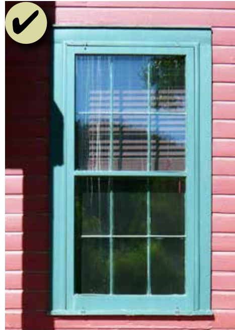
Figure 89: Use storm windows designed to match the historic window frame if placed externally.
