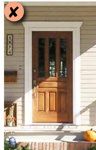
Figure 96: This three-pane replacement door is not typical for most of the historic styles located within the neighborhoods. A simple single-pane window door should be used instead.
