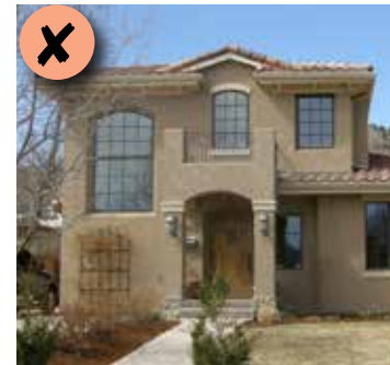
Figure 128: This building is not compatible with the Old Town Neighborhoods. Its windows and entry features are out of proportion with others in the context. It is also too wide.
