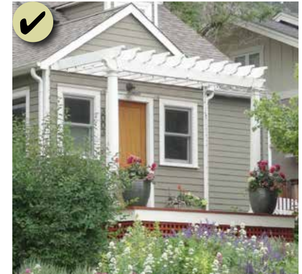
Figure 155: The addition of a trellis on a simple vernacular building at the porch stoop is appropriate.
