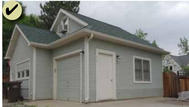
Figure 178: Use materials that are of a similar color, texture and scale to materials of the primary building.
