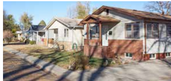
Figure 55: Character Area 6 Row of aligned Minimal Traditional homes with side driveways to parking in the rear
