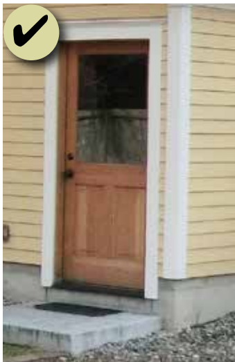
Figure 93: When necessary, a simple wood half glazed door with paneling below is an appropriate replacement door for many of the modest historic styles.
