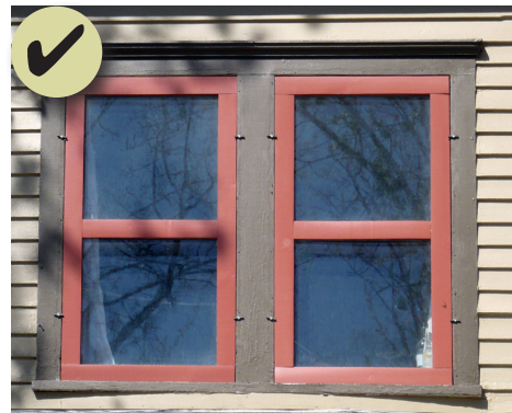
Figure 91: The storm windows match the opening; however, it would be more appropriate if the frames matched the historic window sash similar to the image shown above.
