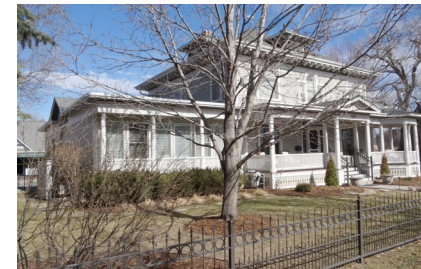
Figure 11: Character Area I Queen Anne with Italianate detailing and addition. In this case, it would have been more appropriate to set back the addition from the front façade.
