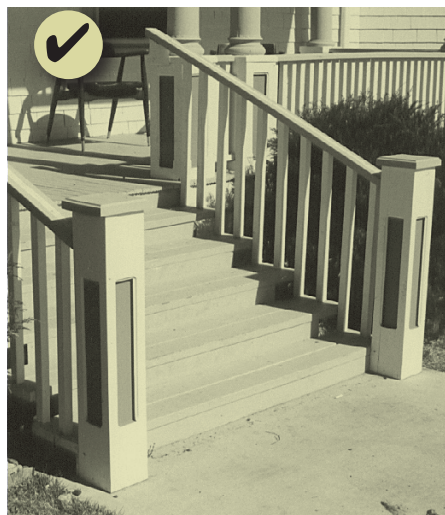
Figure 71: After: Railing has been repaired and the base of the post has been replaced in-kind. This is an appropriate approach.
