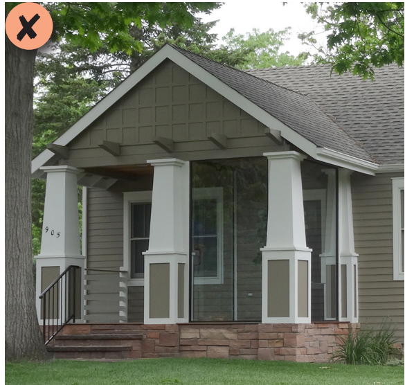
Figure 153: This porch is not in proportion with the historic context since the porch columns are oversized.
