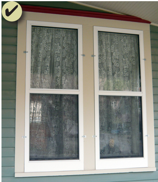
Figure 90: The storm windows match the opening; however, it would be more appropriate if the frames were wood to match the original material.
