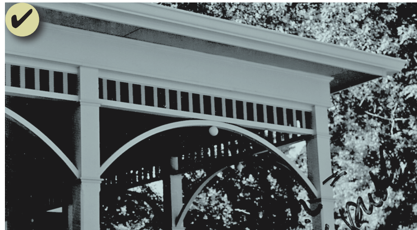
Figure 74: When reconstruction of a historic feature is impossible, develop a new design that is a simplified interpretation of it. This detail in the porch bracketing has simple vertical and horizontal elements rather than the historic curvature detail.
