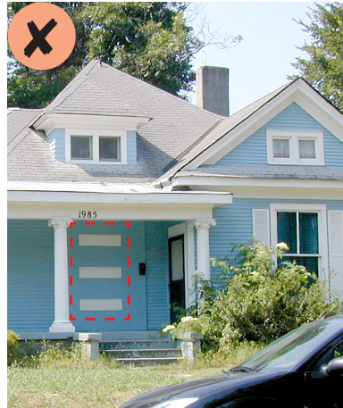
Figure 84: This three pane window alteration is inappropriate and should be restored to its original historic configuration.
