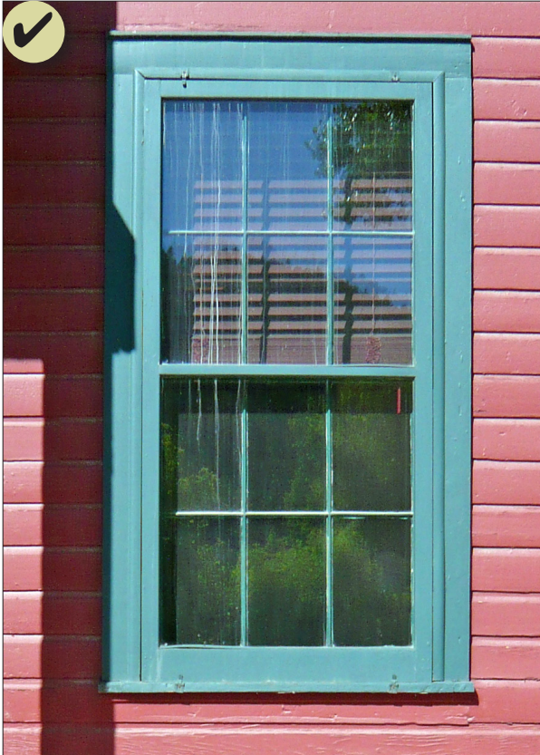
Figure 123: Consider using a storm window to enhance the energy efficiency of an existing historic window, rather than replacing it.
