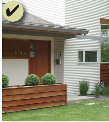
Figure 163: Wood siding is an appropriate material. Note this addition uses a narrow wood lap to differentiate it from the existing building.
