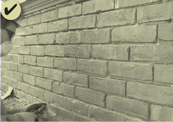
Figure 75: Re-point mortar joints where there is evidence of deterioration. Use correct mortar to prevent problems and match the historic design.
