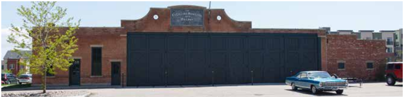
The Fort Collins Car Barn provides an opportunity for an iconic historic structure to be rehabilitated and adapted into a year-round marketplace.
