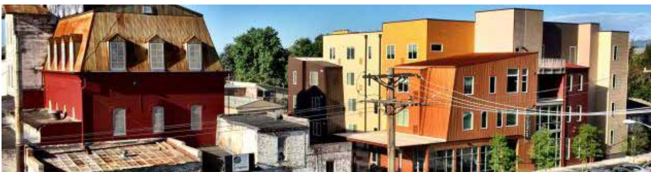
Artspace in Loveland combines a rehabilitated historic mill building with new construction to provide an affordable live/work space for creatives.
