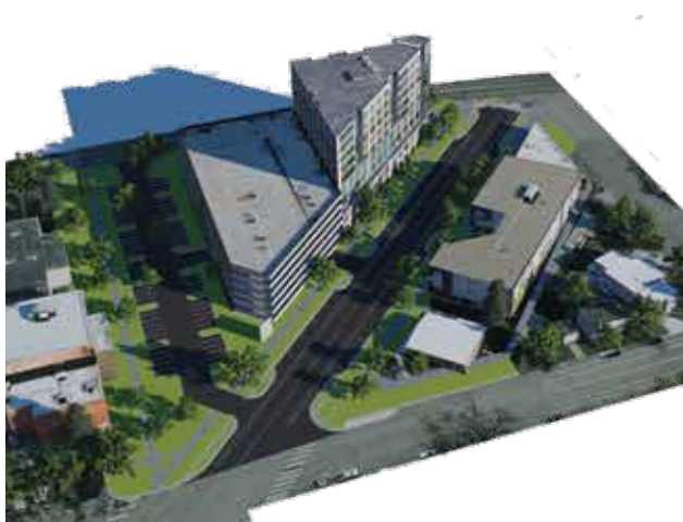
Example of maximized development based on the current height limit on the site and parking requirements—requires a major parking structure
