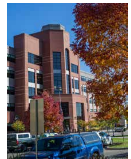
The newly constructed Utilities Administration Building (Laporte and Howes) serves as an aspirational example of 'green building' for energy efficiency.
