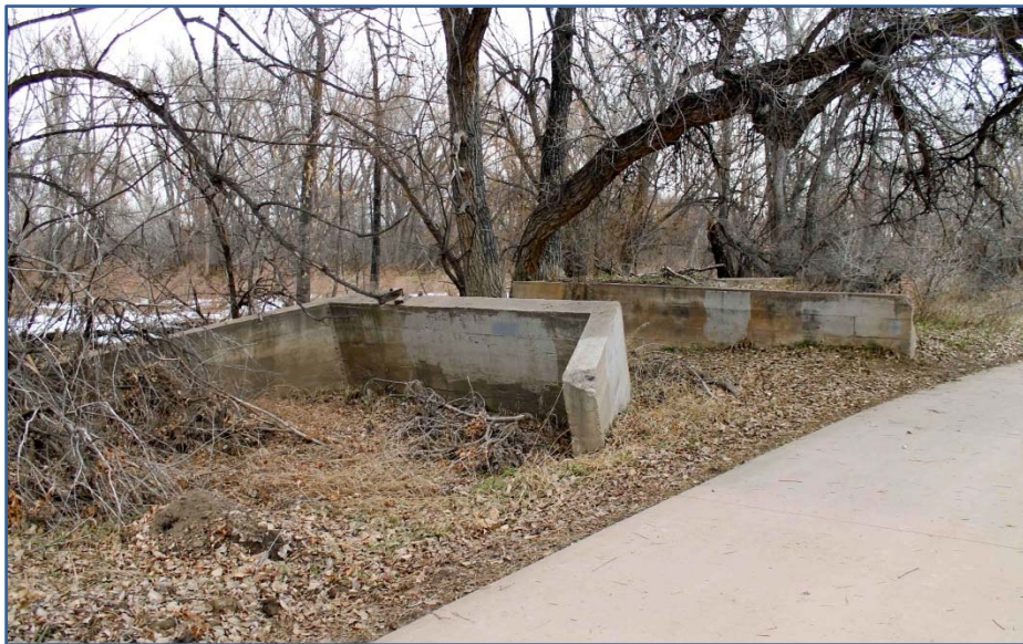
Figure 2.9 Historic Mason & Hottel Mill Race Headgate Structure
