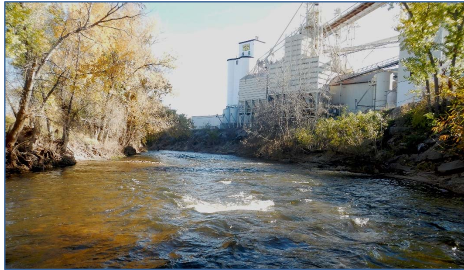
Figure 2.50 Adjacent Industrial Land Use and Concrete Rubble along Southwest Bank
