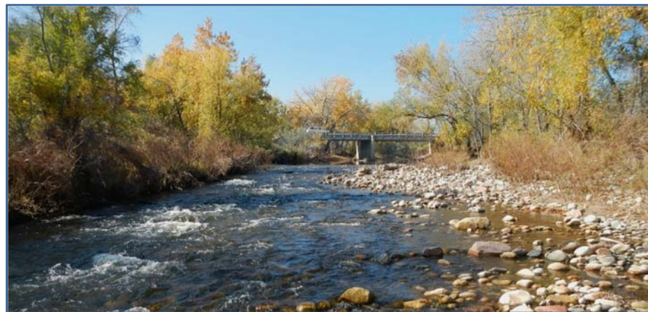
Figure 1.1 Poudre River Looking West to the Shields Street Bridge
