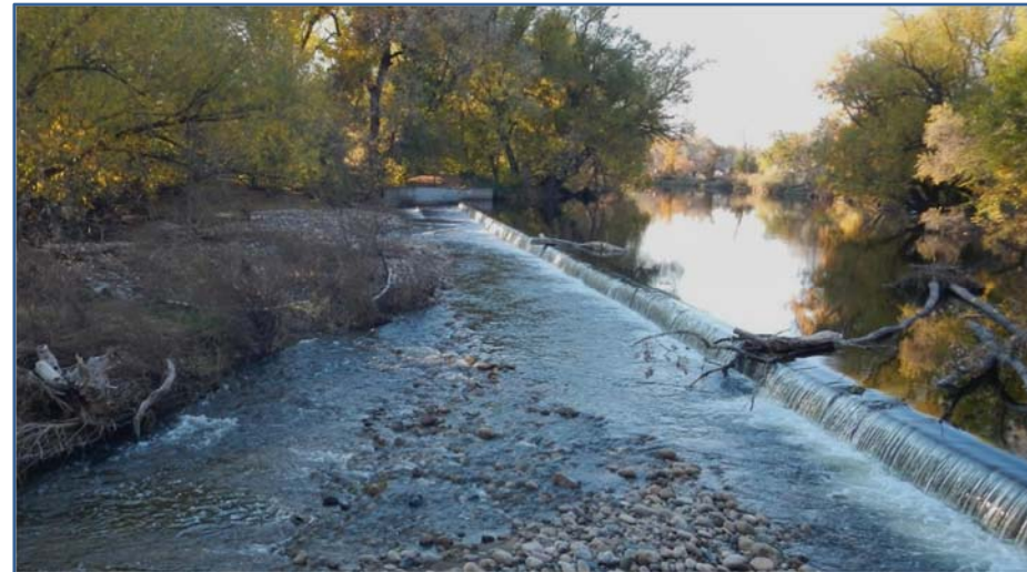
Figure 1.5 Lake Canal Diversion Structure near Lee Martinez Park
