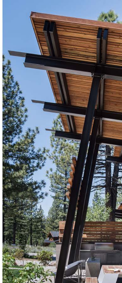
Steel Beams & Wood Decking
