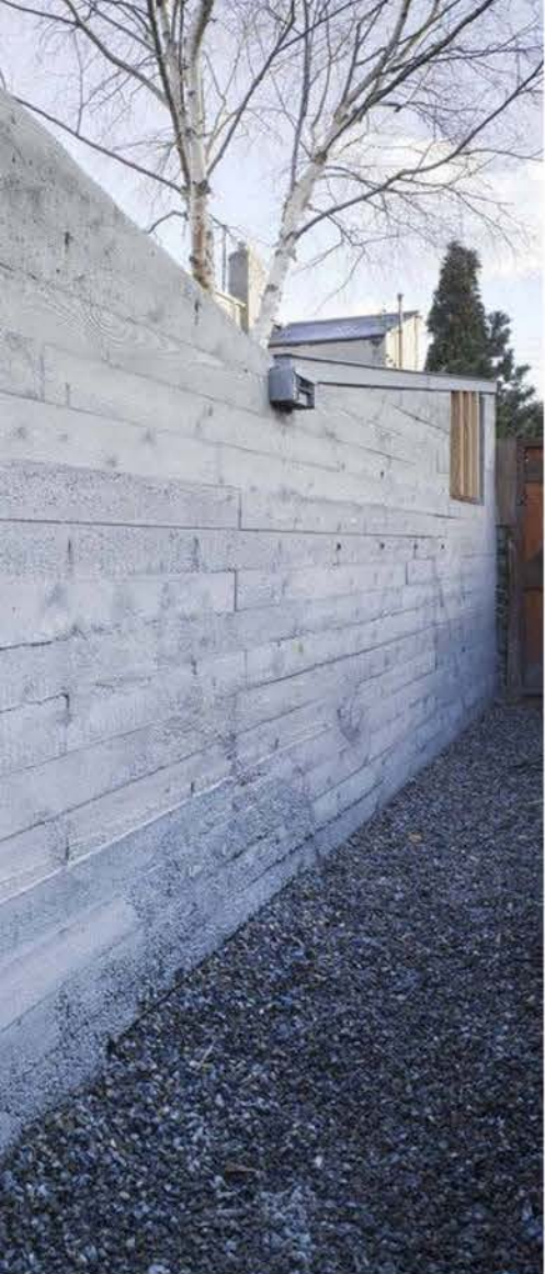
Board Formed Concrete
