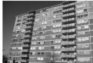
Photo 3: Exposed Frame. The bad news is that we have built lots of these. The good news is that they are easy to fix by recladding them with exterior insulation.
