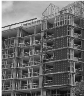
Photo 1 (left): "Harley Davidson" Architecture. The projecting concrete slabs transfer heat across the enclosure. Photo 2 (right): Architectural Statement. Apparently, the projecting slab is visually appealing (who knew?). It catches rain and transfers heat efficiently while wasting floor area (square footage).
