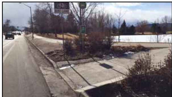
The bus stop adjacent to Rolland Moore Park has accessibility challenges due to the slope of the ramp leading to the bus stop. (Photo credit: Emma Belmont)
