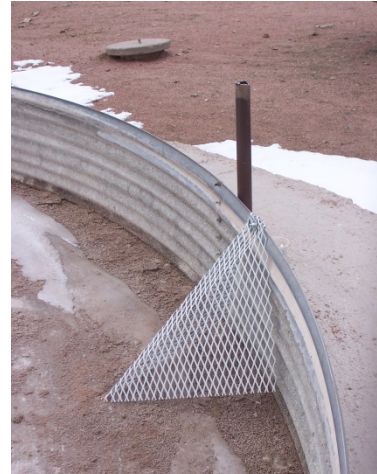
Stock tank escape ladder, installed winter 2006, at Soapstone Prairie Natural Area.
