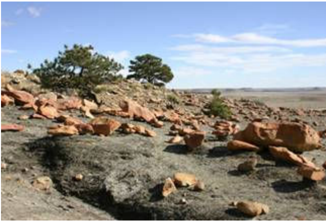
Boulders above the L.R. Camp landslide
