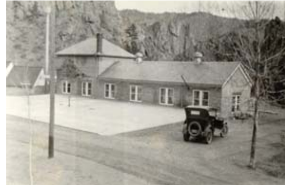
Original treatment plant.
