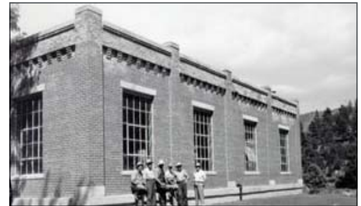
Treatment plant after the last expansion.
