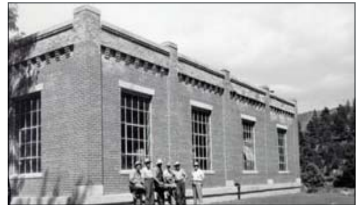
Treatment plant after the last expansion.
