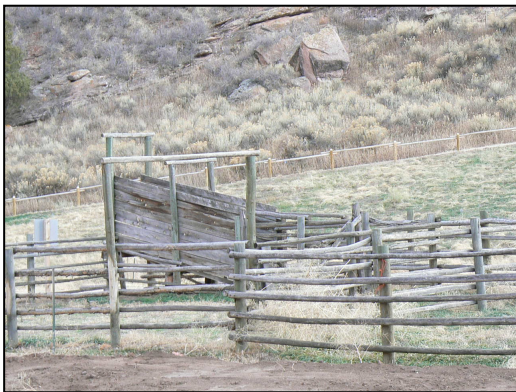
Courtesy of Carol Tunner Figure 103. Cattle chute, December, 2007.
