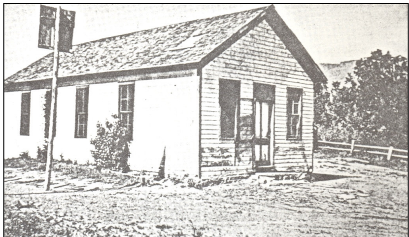
Figure 69. Masonville (formerly Buffum) School built circa 1887.
