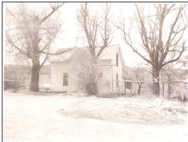
Courtesy of Larimer County Assessor’s Office Figure 97. Hyatt ranch house taken 1981.
