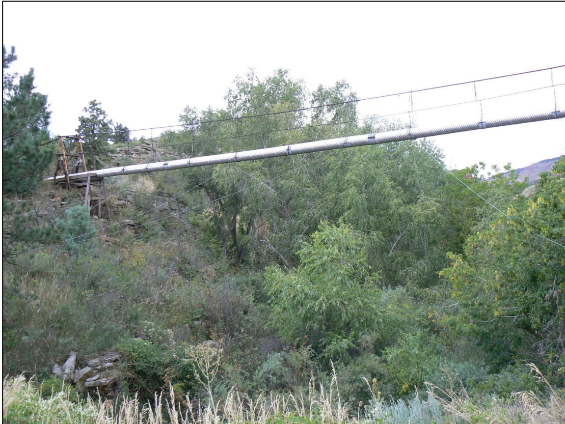
Figure 24. Existing Buffum-Hyatt Ditch closed-siphon pipeline over Brooks Canyon.
